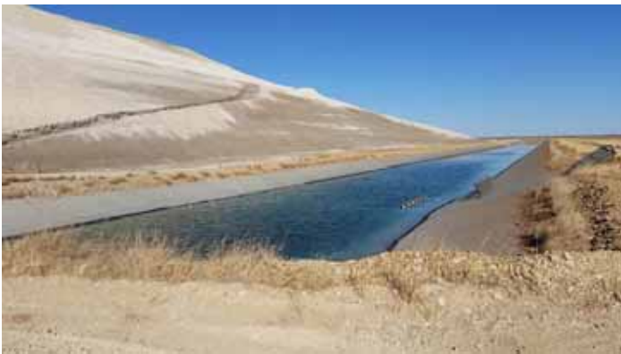
Image 2: North end of Cell 4B gypsum stockpile revealing a lined surge ditch.
