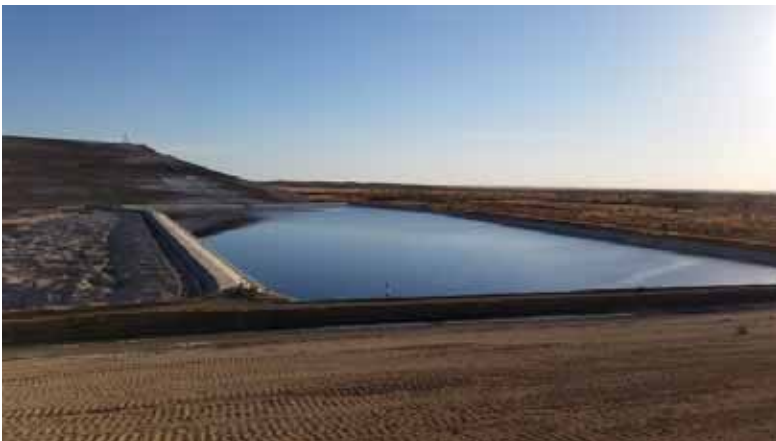
Image 3: Evaporation & Re-slurry Recirculation Pond 3B
