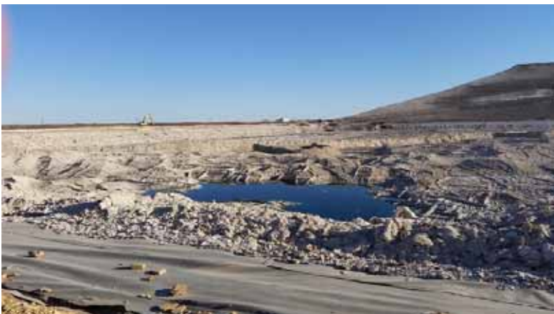
Image 4: Pond 3A dewatered in preparation for geotechnical investigation
