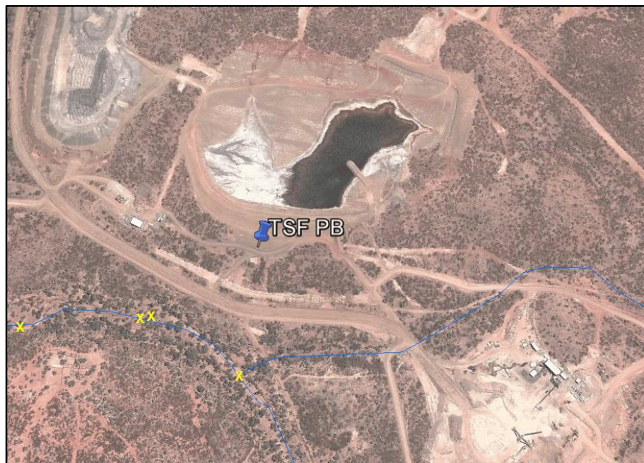
Figure 19 Location of TSF pump-back bore (interception trench). Also, yellow “x” markers depict the locations of where [possible] TSF solution was observed to be seeping to the Coppermine Creek.
