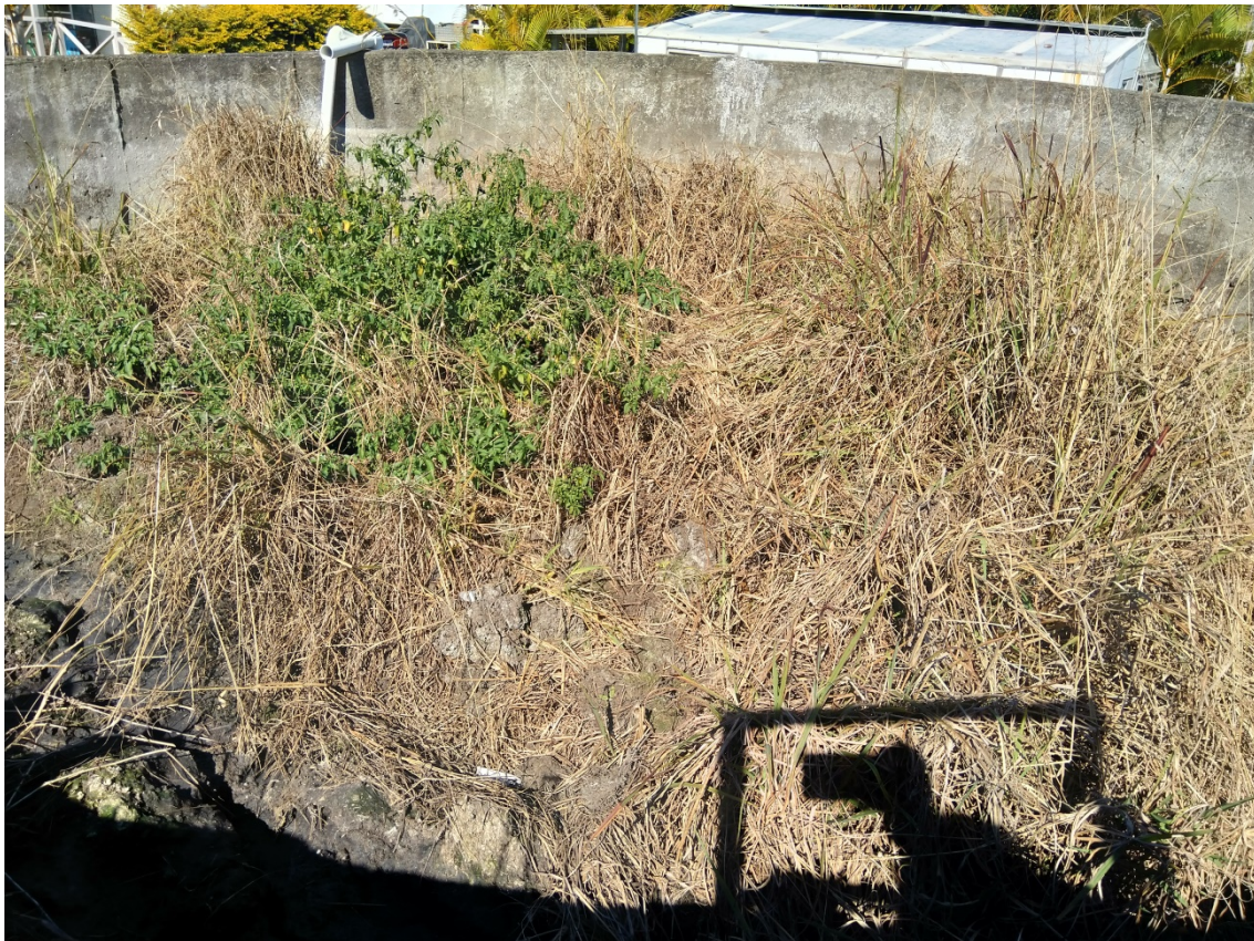
Figure 6: Digester “Scum” Layer
