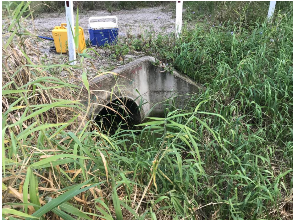
Figure 16 Stormwater Outlet Sample point west of Lot 9/RP230529
