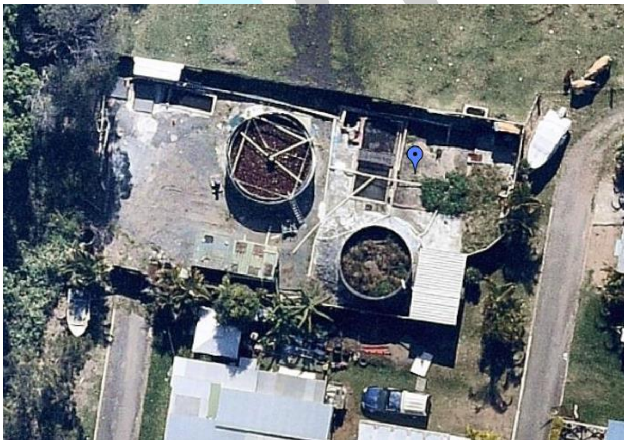
Figure 31 Dried Sludge Disposal Area within STP Compound
