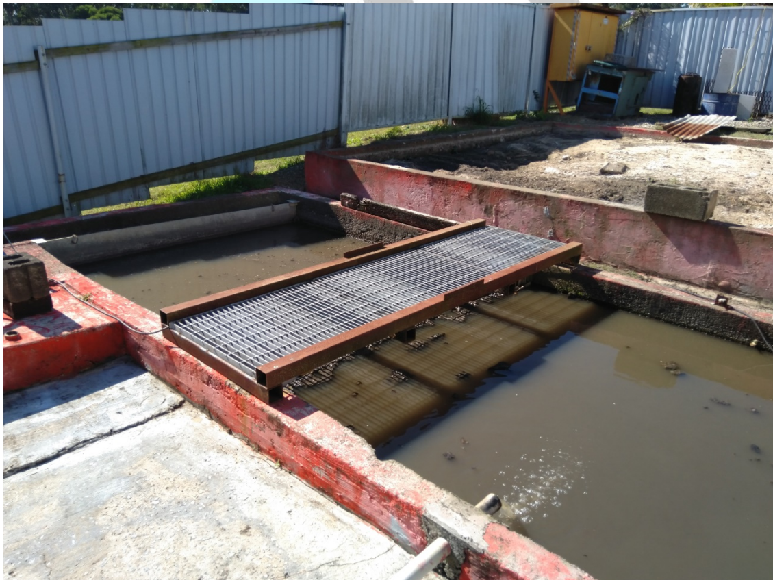
Figure 8: Primary Clarifier Tank Cell 1 (baffle wall located under bridge)
