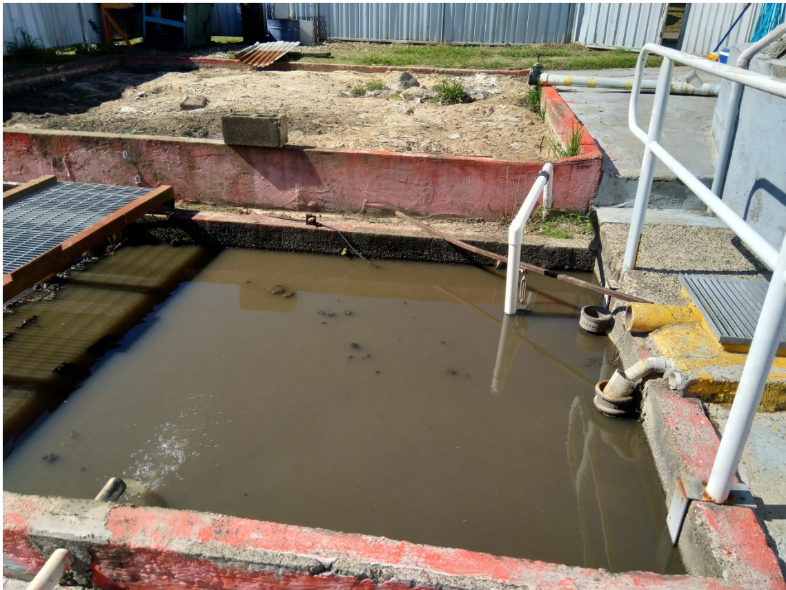
Figure 7 Primary Clarifier Tank – Cell 1
