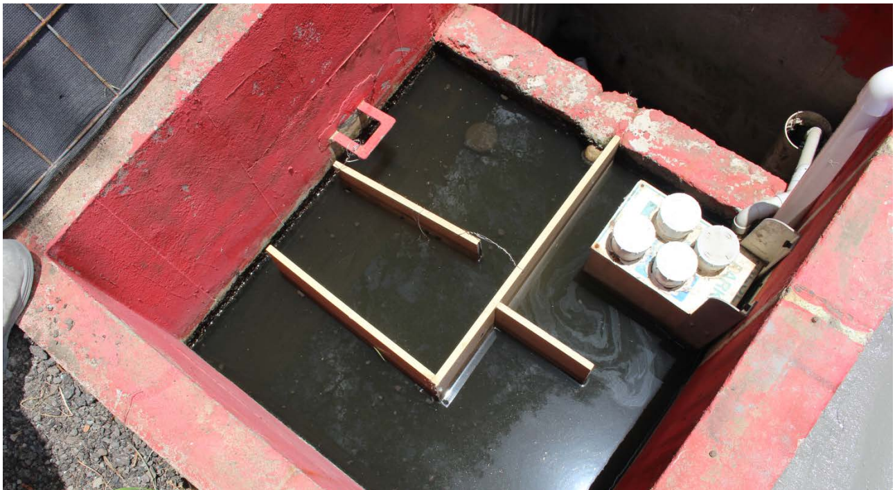
Figure 5: Chlorine Contact Tank Baffling
