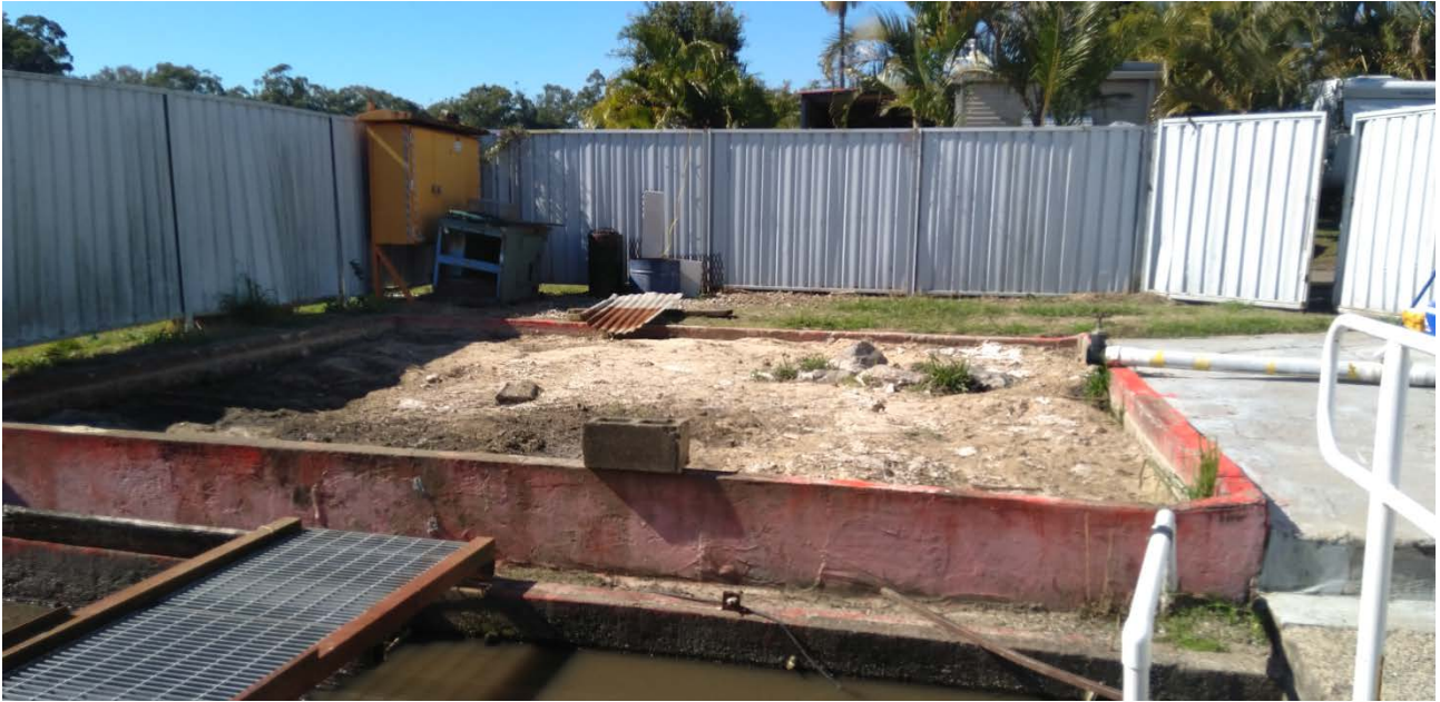
Figure 22: Sludge Drying Bed
