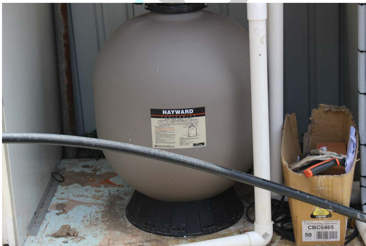
Figure 3: Pressure Sand Filter
