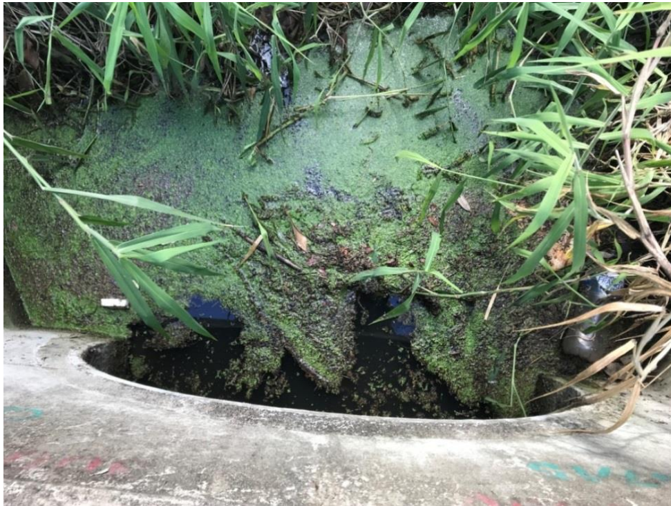
Figure 20 Surface floating vegetation at Stormwater Outlet
