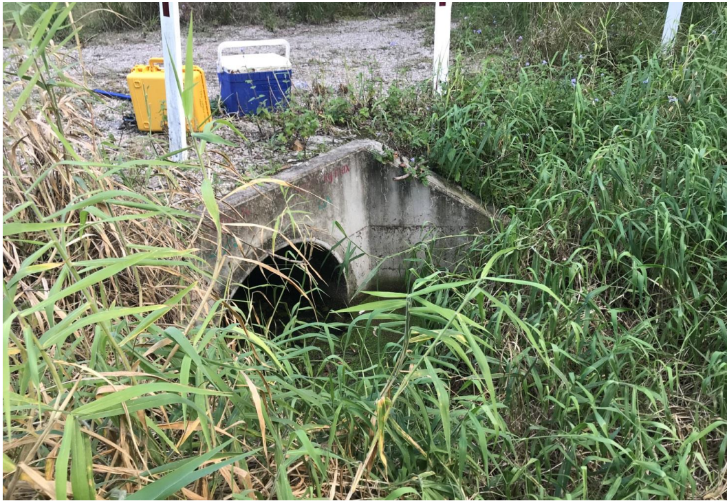
Figure 28 Stormwater Outlet at the ‘tributary of Coolnwynpin Creek’
