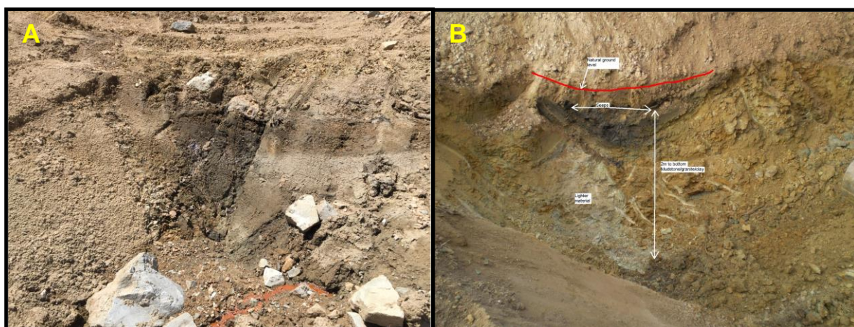
Figure 12: Groundwater seepage downgradient of MRMB10 13
