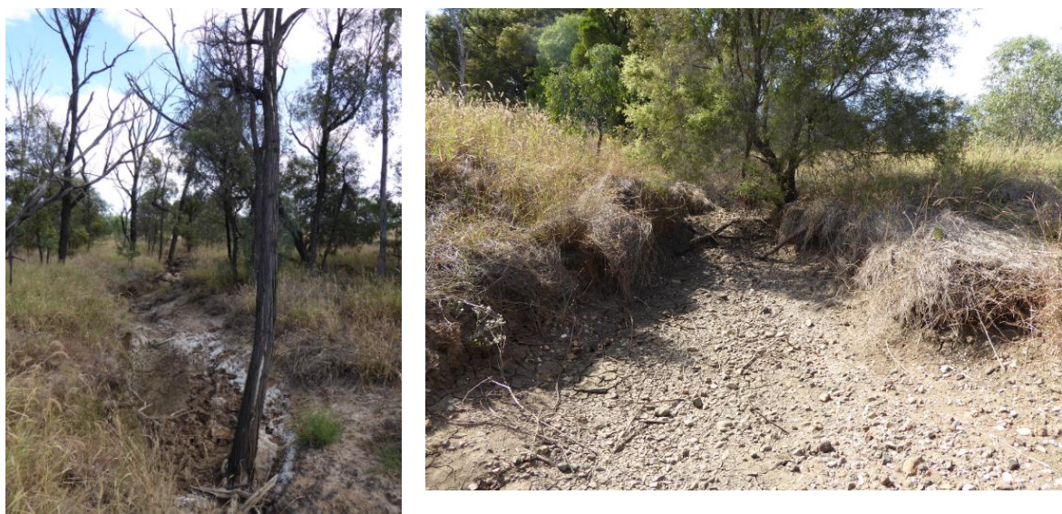
Figure 4.5 (L to R) Standing Dead Trees within the Rock Hole Gully Creek Upstream of the initial ML5656 Mining Lease Boundary (29/06/2017), Rock Hole Gully Creek Downstream Monitoring Location (29/06/2017)
