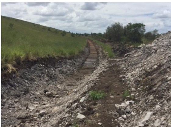
Figure 5.1 Southern Drain (Looking East) (22/11/2017)
