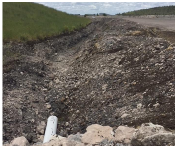
Figure 5.3 Southern Drain Approaching Pipe Culvert at the Western Dump Toe (Looking South) (22/11/2017)
