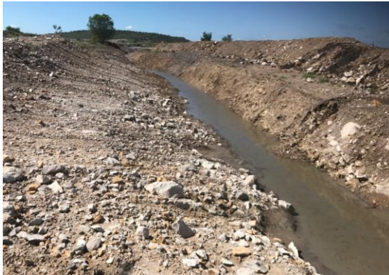
Figure 5.5 Western Drain (Looking North) (25/10/2017)
