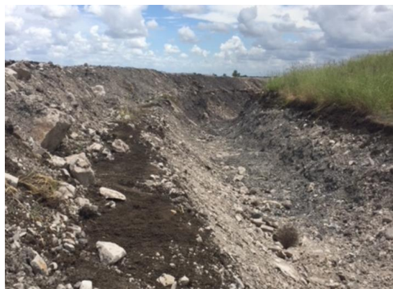
Figure 5.2 Southern Drain Approaching South-West Corner (Looking West) (22/11/2017)
