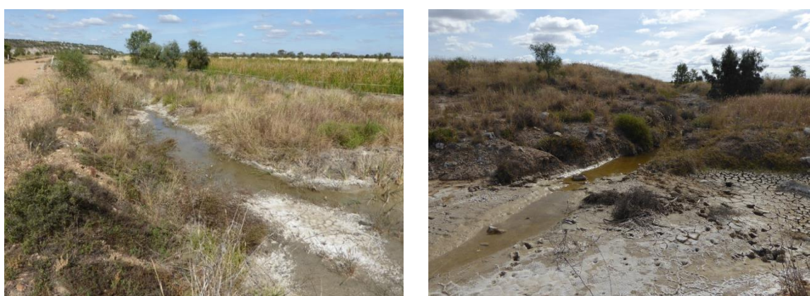
Figure 1.2 (L to R) Seepage Water in Erosion and Sediment Control Drain (29/06/2017), Erosion and Sediment Control Drain Confluence with Clean Water Drain (29/06/2017)
