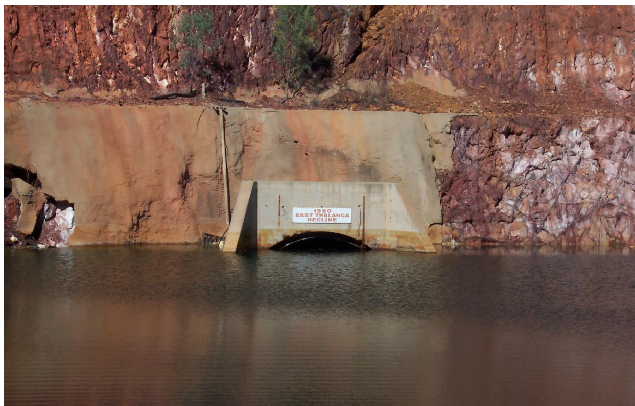
Figure 23 Flooded East Thalanga decline within the Central Pit in 2006. Flood level at approximately RL 308m, inferred from a comparison between mine plans and available topographic maps
