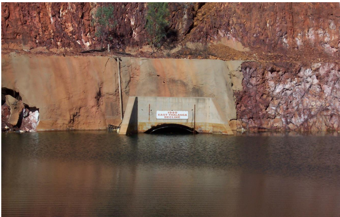
Figure 17 Flooded East Thalanga decline within the Central Pit in 2006. Flood level at approximately RL 308m, inferred from a comparison between mine plans and available topographic maps
