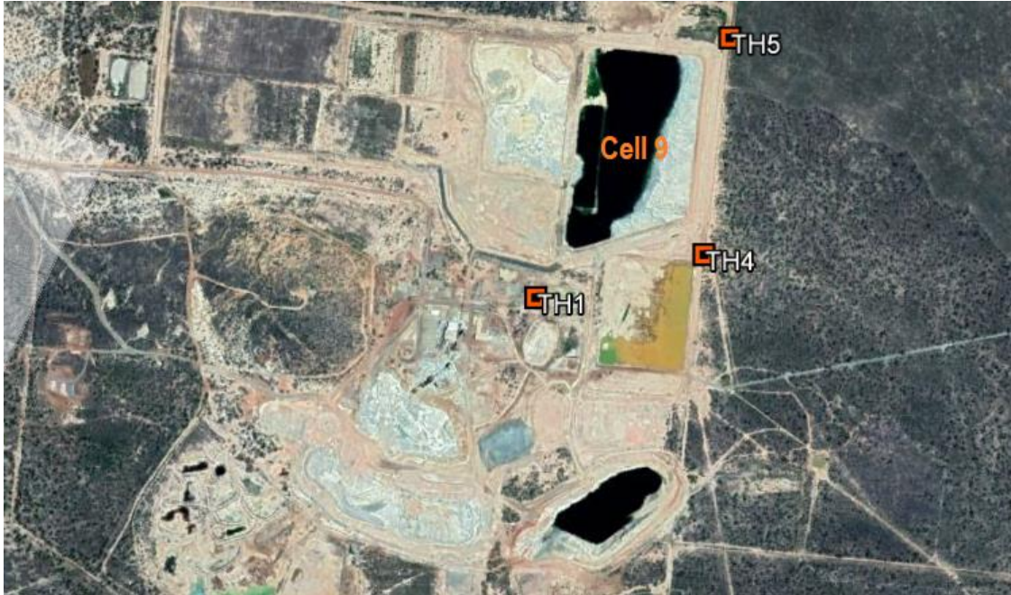
Figure 20 Location of TH1, TH4 and TH5 (installed in 2008) with regards to tailings cell 9
