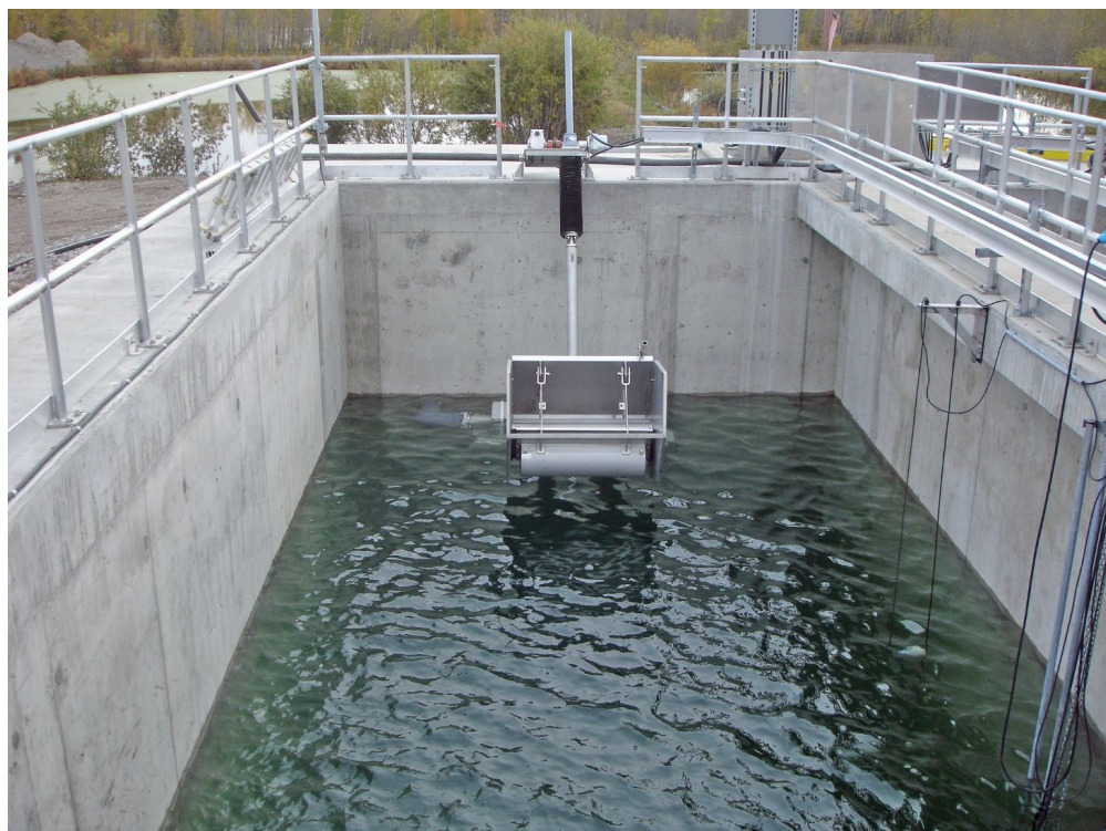
Figure 4: Typical SBR with decanter shown
