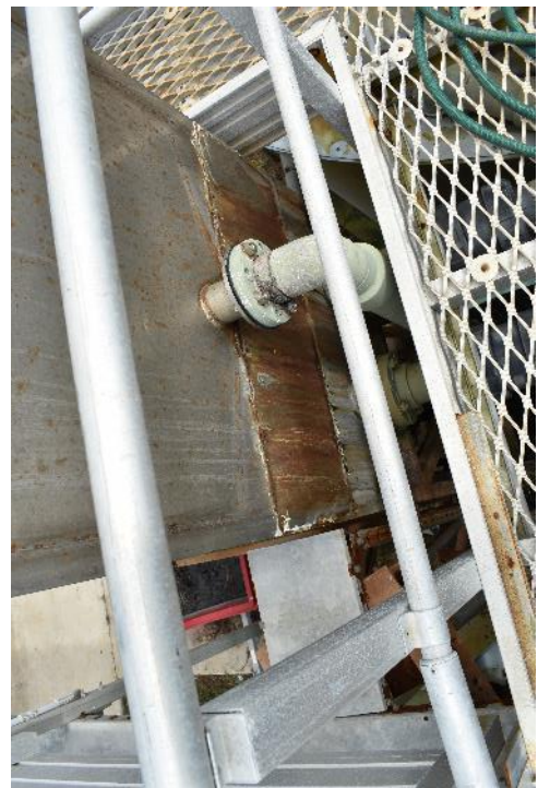
Figure 8 – Inlet Works Area
