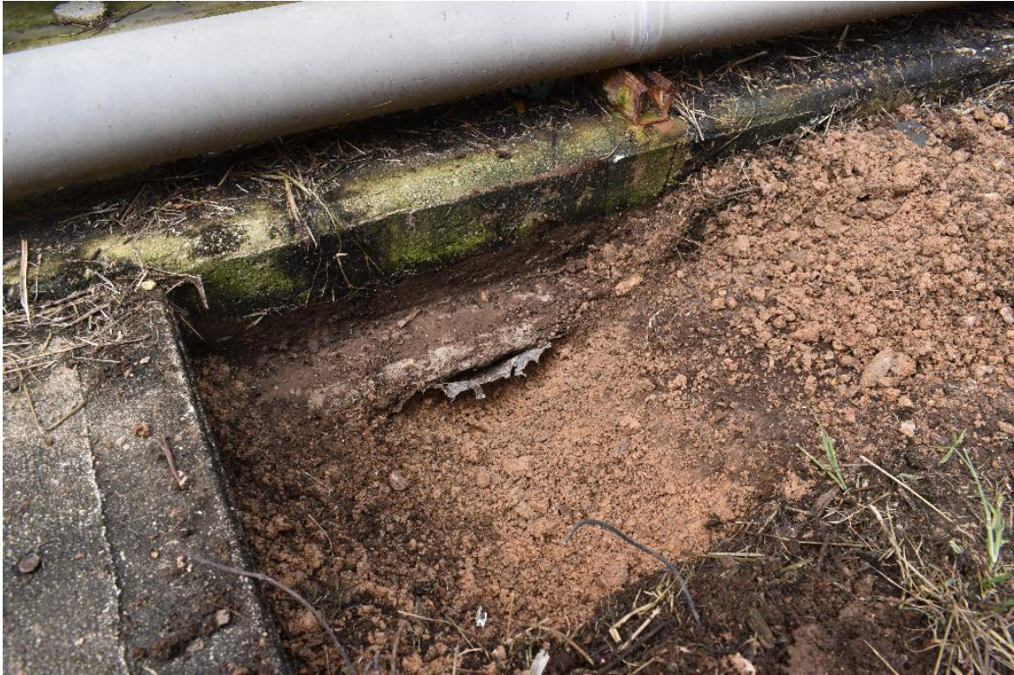
Figure 38 - STP Concrete Slab
