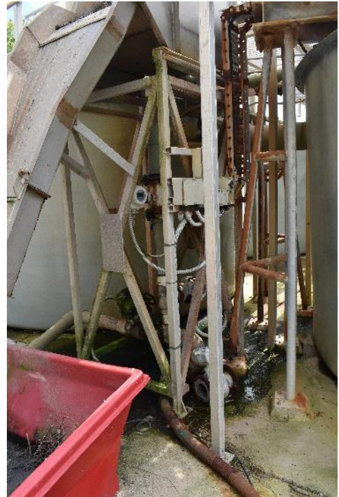
Figure 6 – Inlet Works Area
