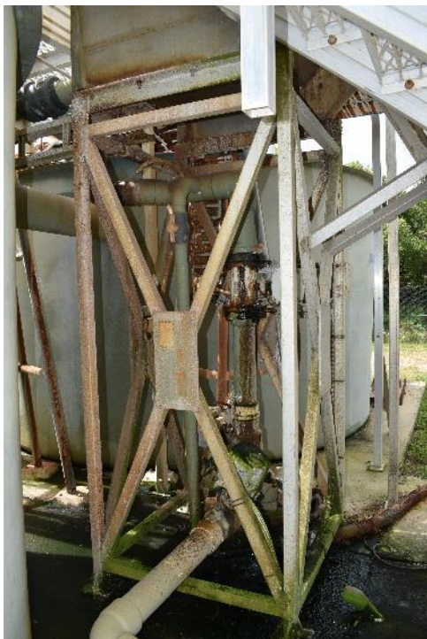
Figure 7 – Inlet Works Area
