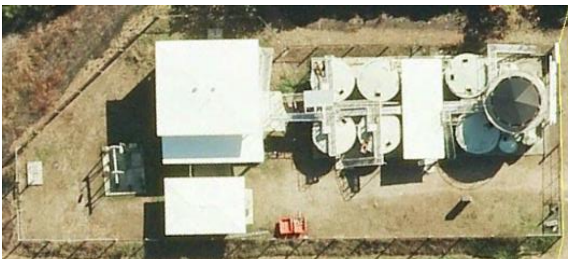
Figure 2 – Aerial view of the existing STP
