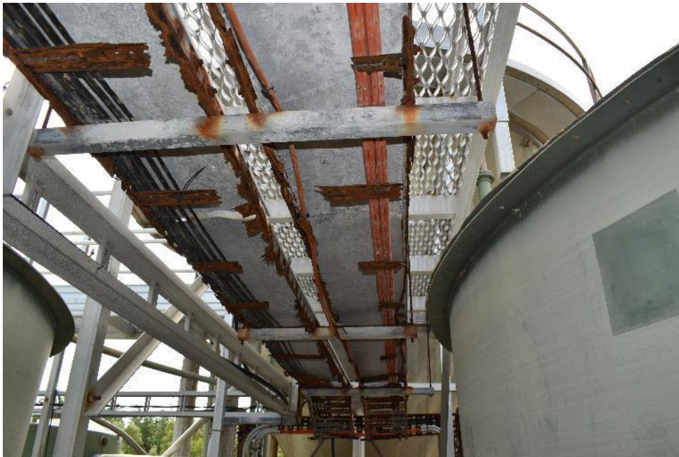
Figure 35 - Severely Corroded Cable Trays
