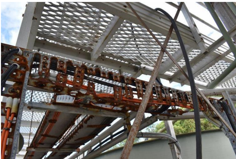
Figure 35 - Severely Corroded Cable Trays
