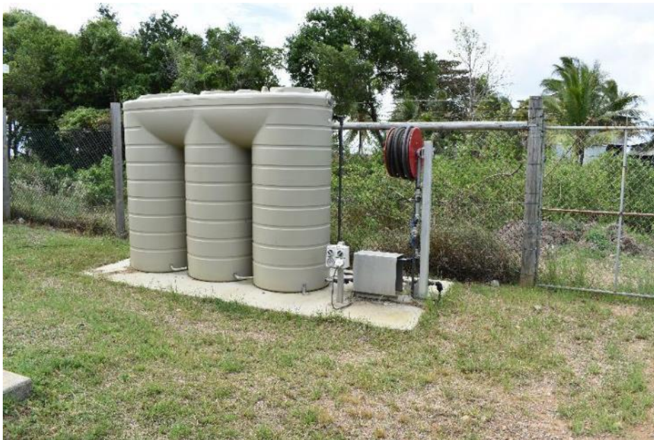
Figure 15 - SPS 1 Service Water System
