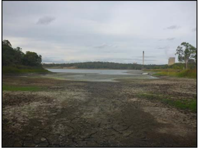
Photo 7.6 Low water level at Meandu Creek Dam
