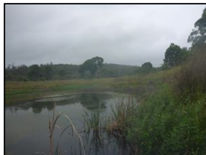
Dam (south facing):
