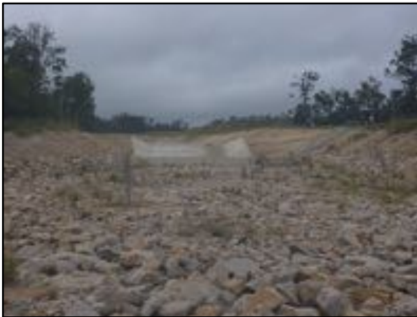
Figure 6.5 Highly modified diversion channel at Black Creek site BC2
