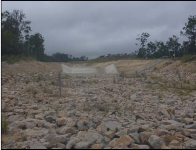
Photo 7.5 Highly modified diversion channel at Black Creek site BC2
