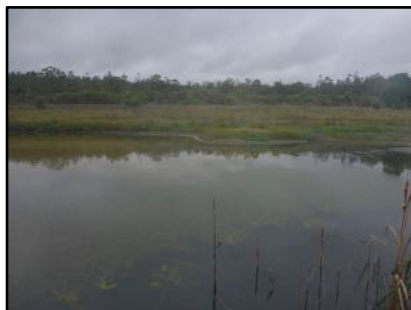
Dam (north facing):
