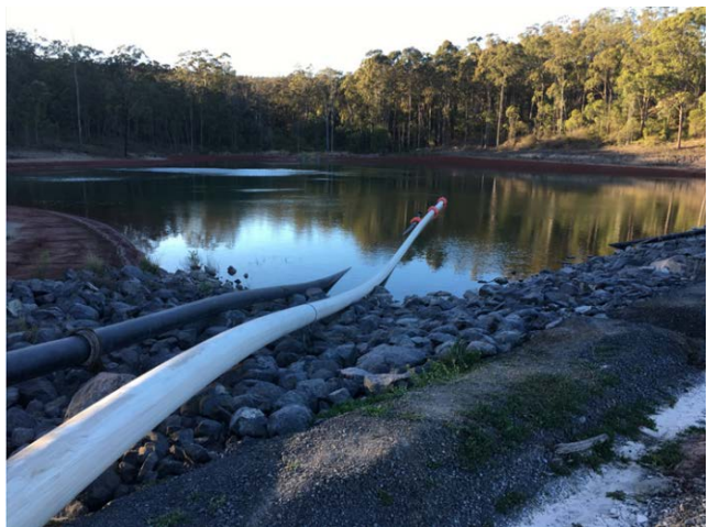
Photo 2.6 Pipeline in RD26
