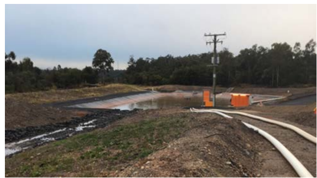
Photo 2.8 RD27 at completion
