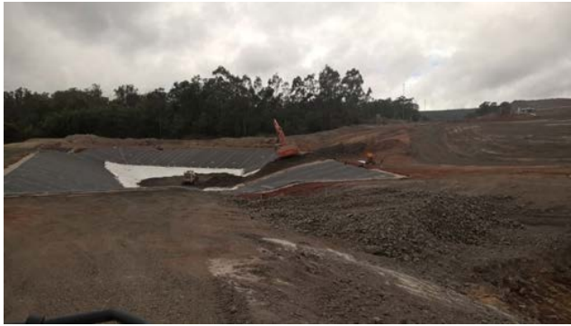
Photo 2.7 RD27 during construction
