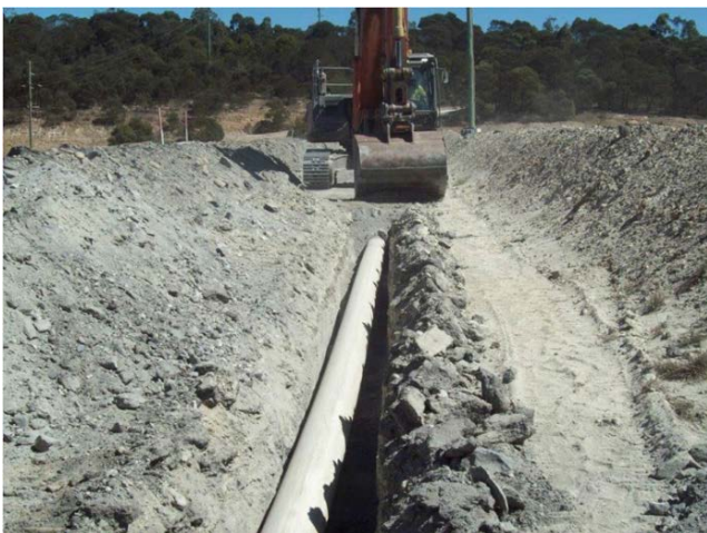
Photo 2.5 Construction of pipework
