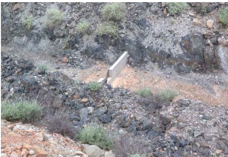
Figure 5-27: BSOC WRD Weir 2 after construction (January, 2016)
