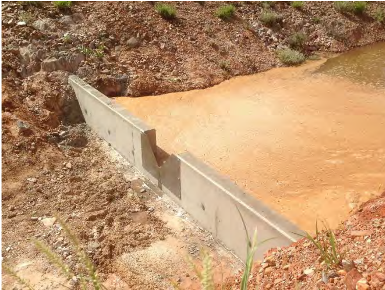
Figure 5-28: BSOC WRD Weir 3 after construction (January, 2016)
