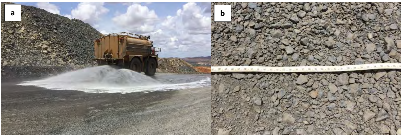
Figure 5-24: Infiltration observations on highly trafficked / compacted area. a) water infiltration test, b) compacted waste rock surface (December, 2015)
