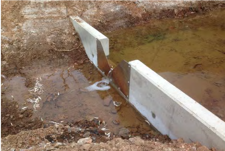
Figure 5-26: BSOC WRD Weir 1 after construction (January, 2016)
