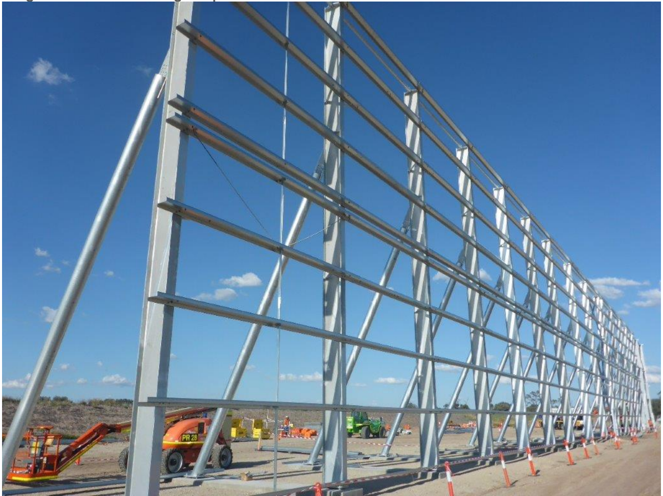
Image 1 - Steelwork nearing completion on Northern Barrier Section
