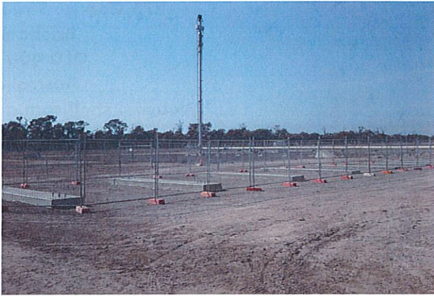
Images 3 – Completed Pile Caps adjacent to Pond Wall
