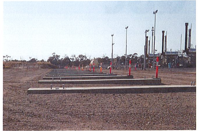
Image 1 & 2 – Completed Pile Caps – Eastern Extent and Northern Extent
