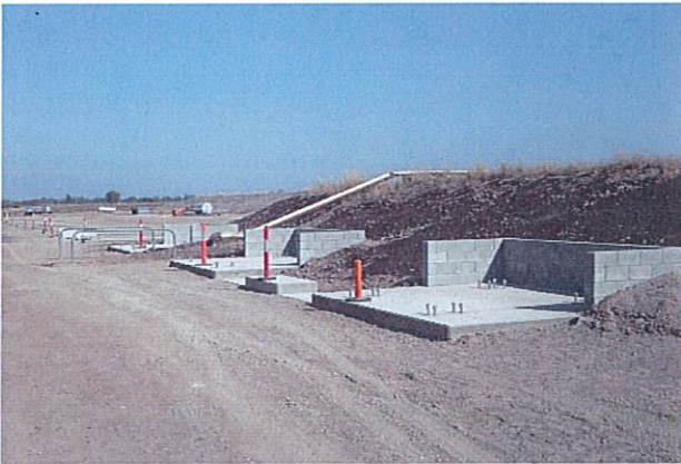
Images 3 – Completed Pile Caps adjacent to Pond Wall
