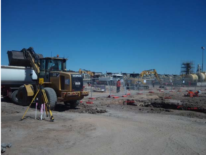
Image 1 – Excavating Pile Caps
