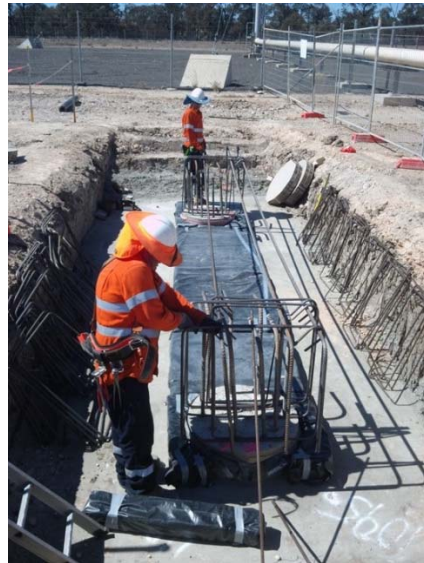
Image 2 – Binding the Piles
