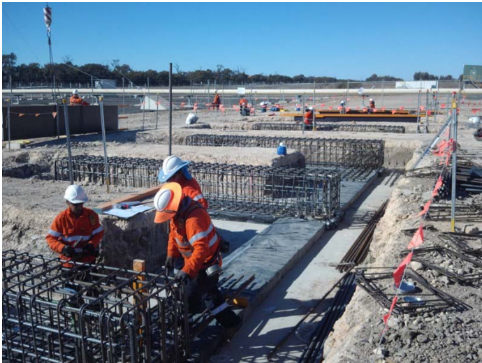
Images 3 & 4 – Overview of Works On Site
