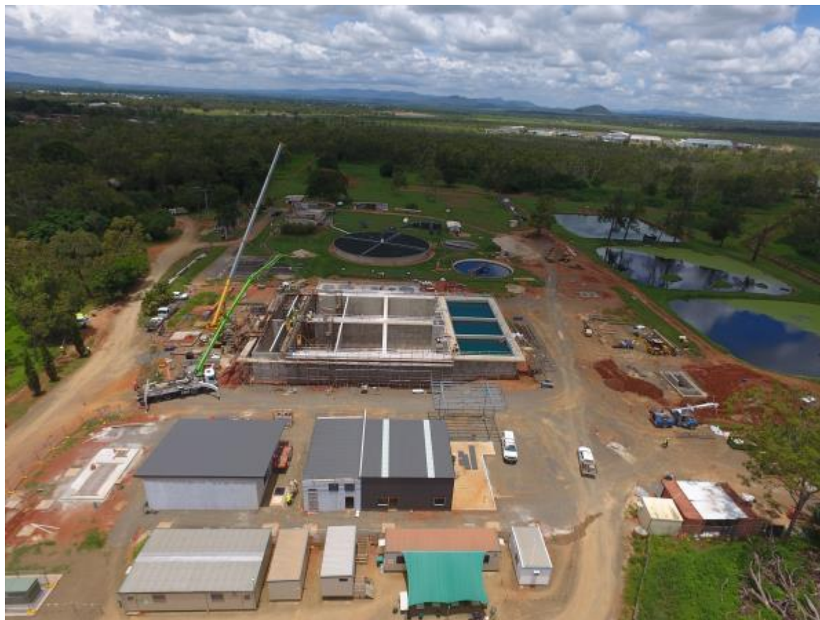
Photo 1: Aerial photo of Mareeba WWTP construction.
