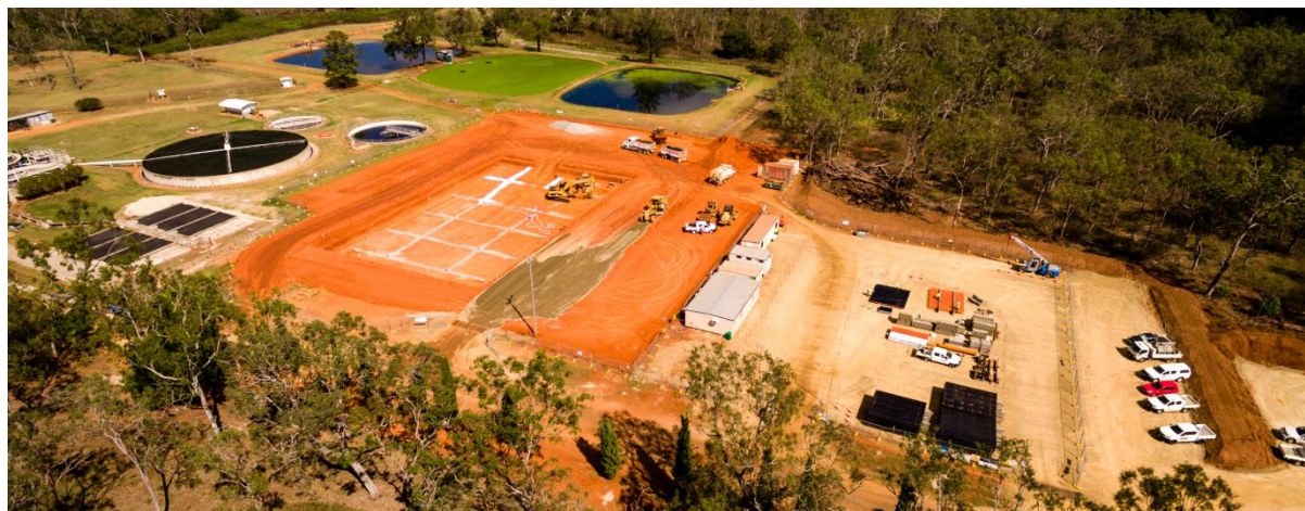
Photo 1: Aerial photo of Mareeba WWTP construction.
