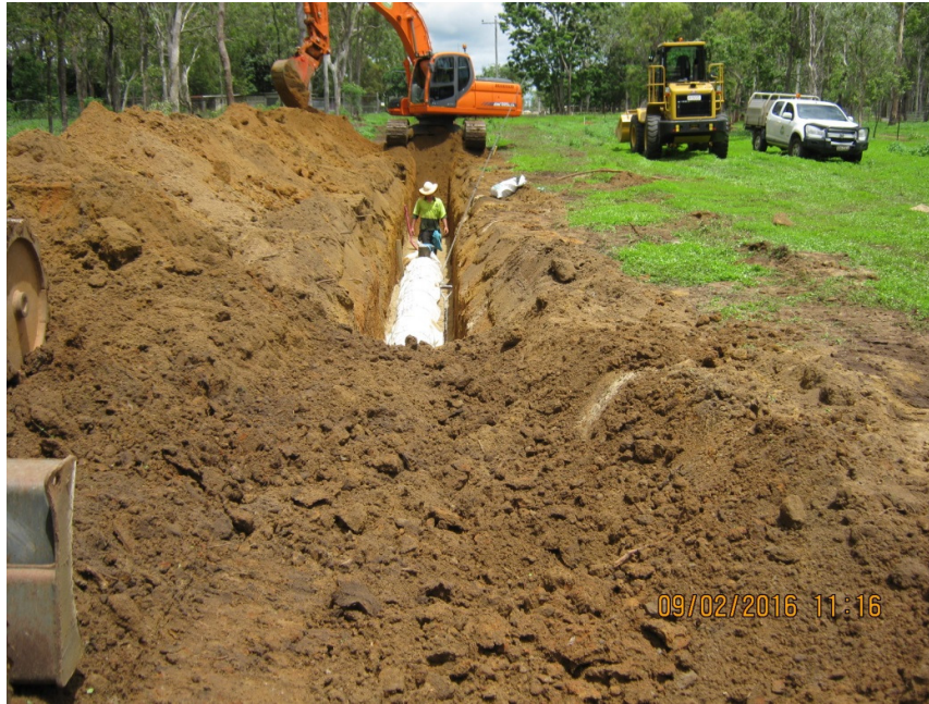
Photo 1 - Installation of the new rising main to the Mareeba Wastewater Treatment Plant is nearing practical completion.
