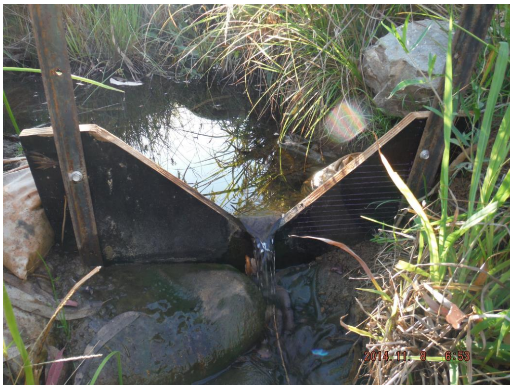
Photograph of v-notch weir at 8 th November 2014
