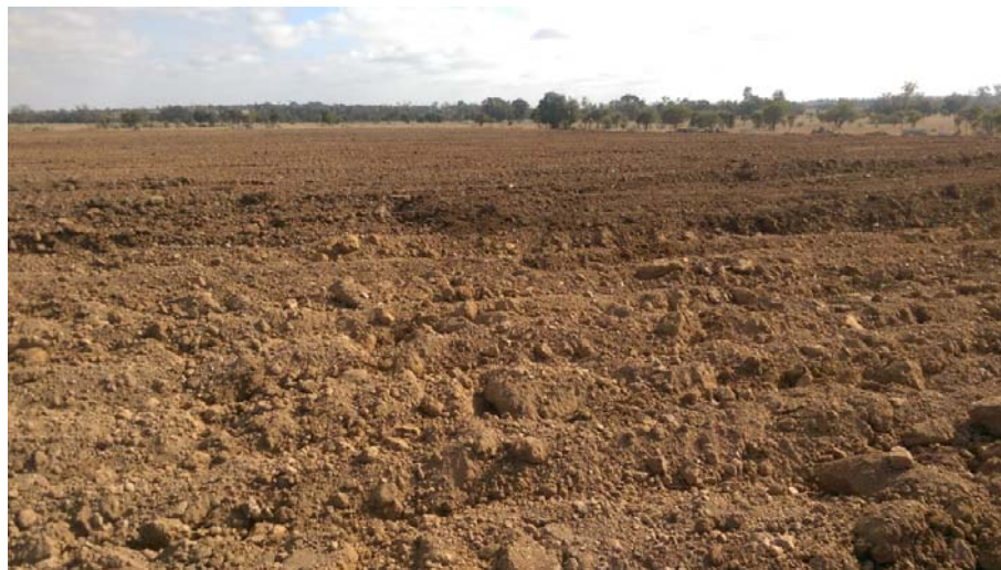
Figure 19 Spreading the topsoil over the ripped subsoil during rehabilitation of the Dawson dam
