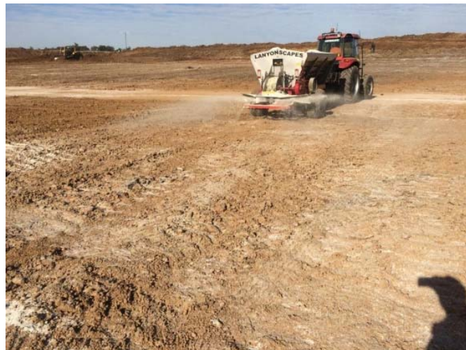
Figure 14 Spreading gypsum onto the reformed basement layer after completion of the mix and bury process
