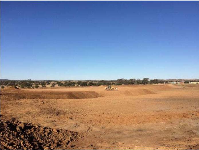
Figure 17 Spreading the subsoil over the reformed dam basement
