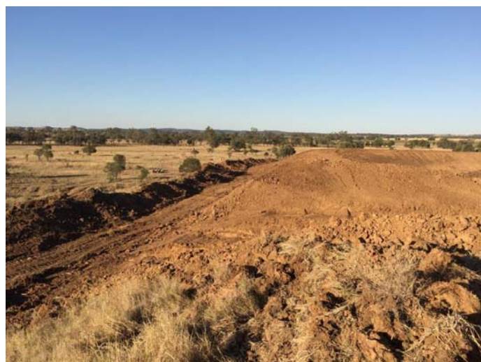
Figure 16 Topsoil that had been scraped of the outside of the dam walls and stockpiled temporarily
