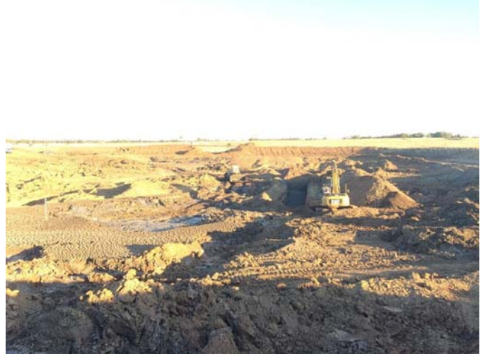
b) Pits and stockpiled material that has been excavated
