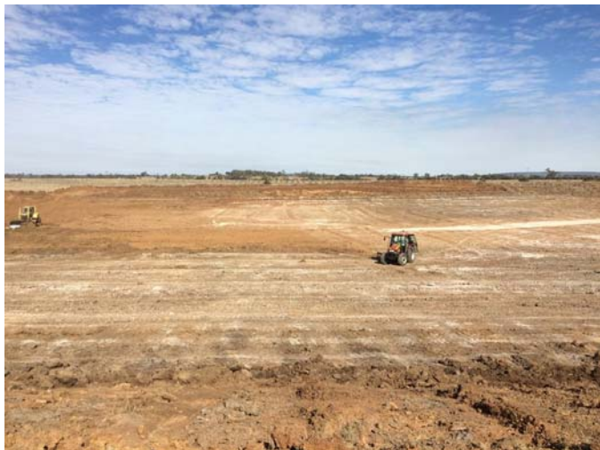
Figure 14 Spreading gypsum onto the reformed basement layer after completion of the mix and bury process
