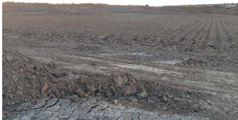
Figure 18 Deep ripping the subsoil to a depth of 1m
