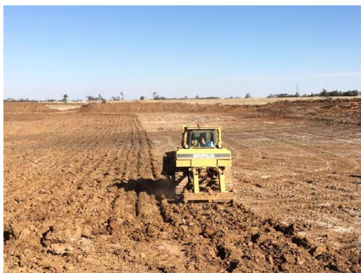
Figure 15 Ripping the reformed basement layer formed after the mix and bury process
