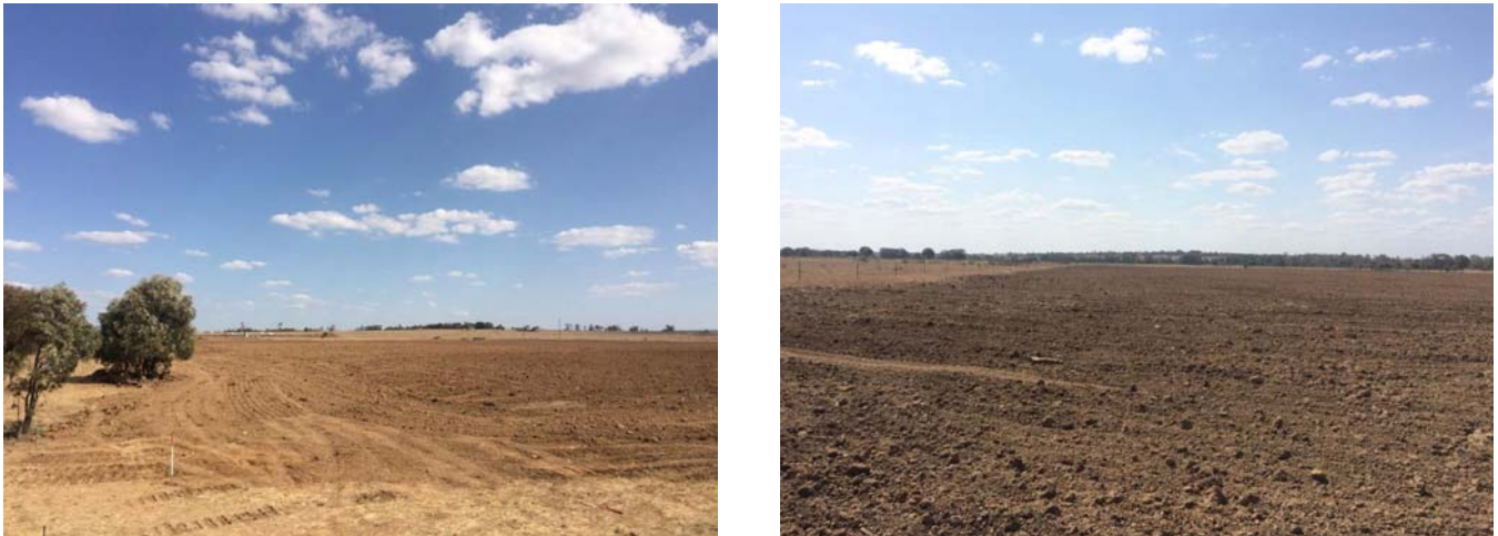
Figure 21 The finished surface after the rehabilitation earthworks were completed
