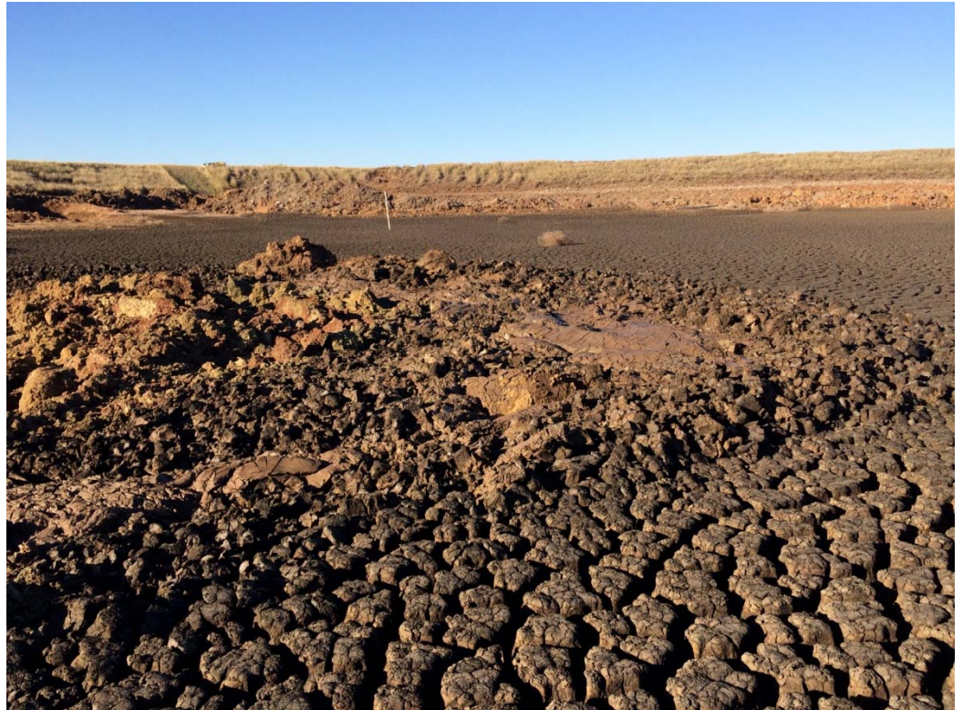
Figure 2 General views of the Dawson Dam site before rehabilitation started
