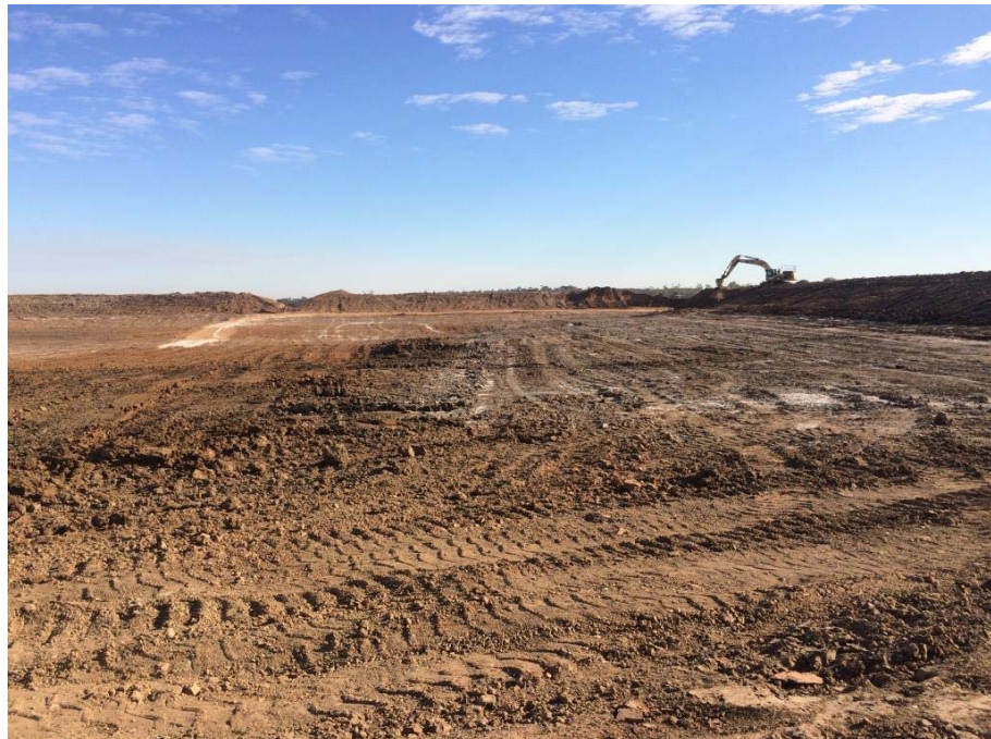
Figure 13 Reformed basement surface after the mix and bury process was completed
