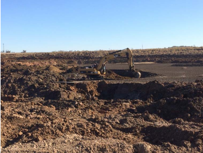
a) A pit being excavated during the mix and bury process
