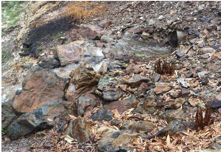
Figure 1 – Significant volume of stormwater entering the contaminated stormwater pond (significant roof stormwater)
