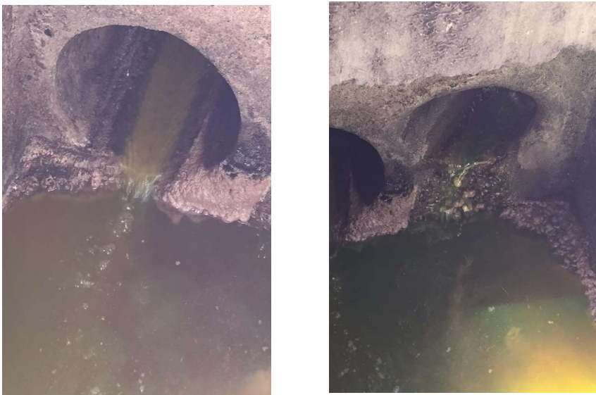
Figure 8 & 9 – Contaminated Streams entering Drain 1 identified with dye (to be diverted to WWTP)
