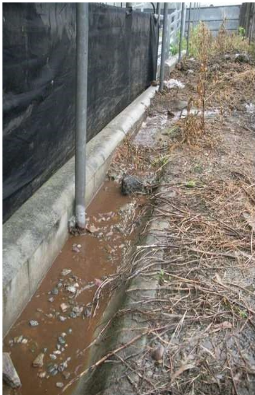
Figure 3 (left) & 4 (right) – Contaminated run-off from holding pens entering roofed stormwater
