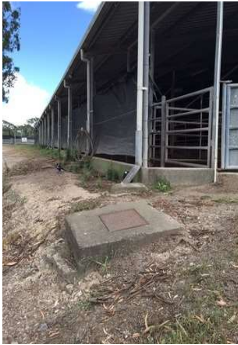
Figure 2 – Roofed Stormwater drainage system on southern side of roofed cattle pens
