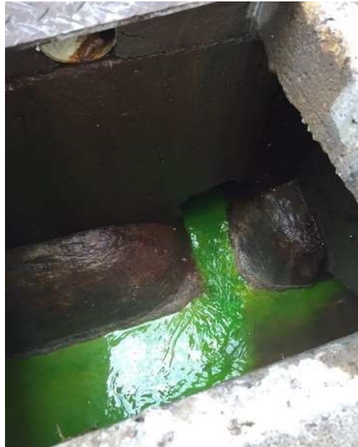
Figure 10 – Roof Stormwater from Kill Floor Roof entering Drain 2.
