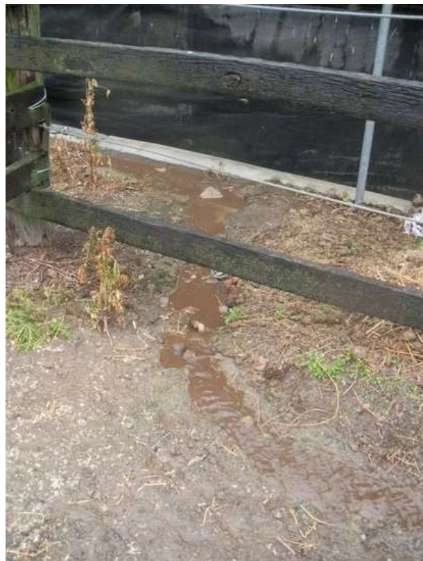
Figure 3 (left) & 4 (right) – Contaminated run-off from holding pens entering roofed stormwater
