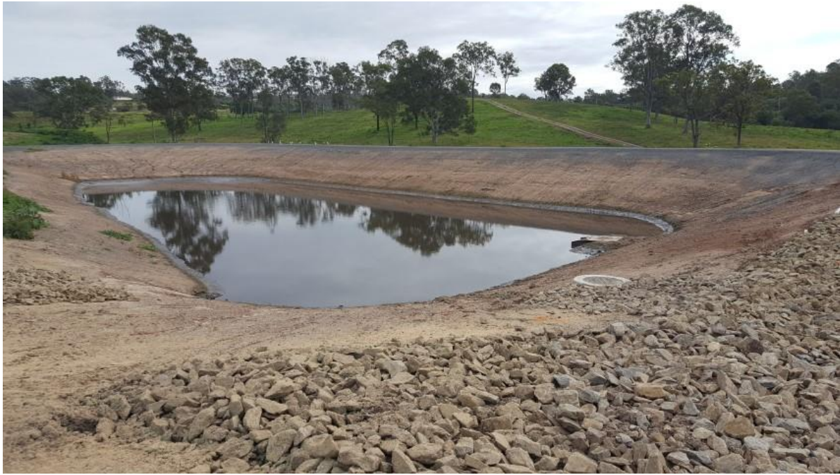
Figure 2: The completed Western Contaminated Stormwater Pond.
