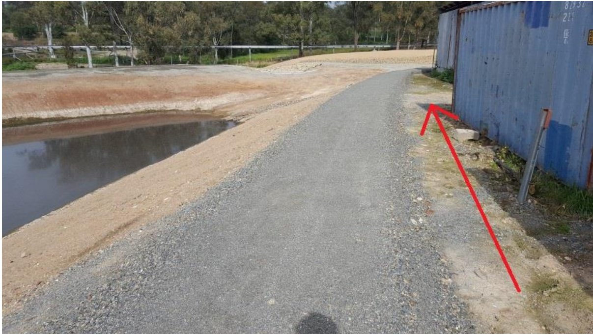
Figure 3: Clean stormwater is directed along the topside of the eastern contaminated pond to the creek.
