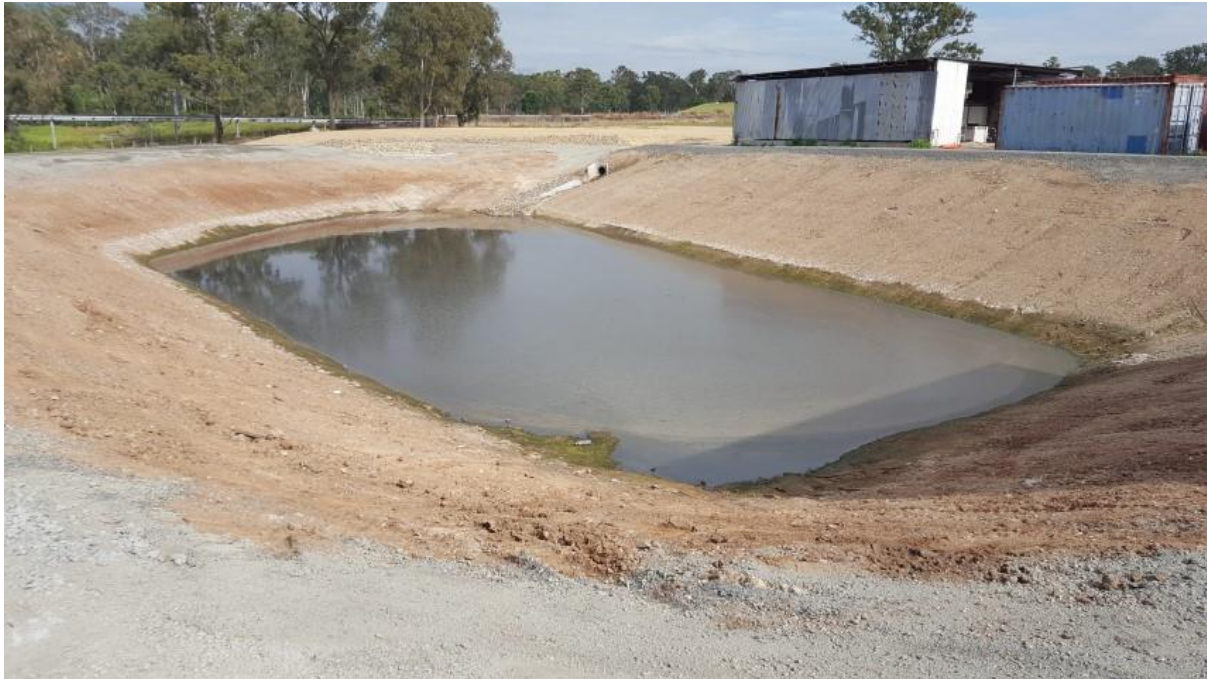
Figure 1: The completed Eastern Contaminated Stormwater Pond
