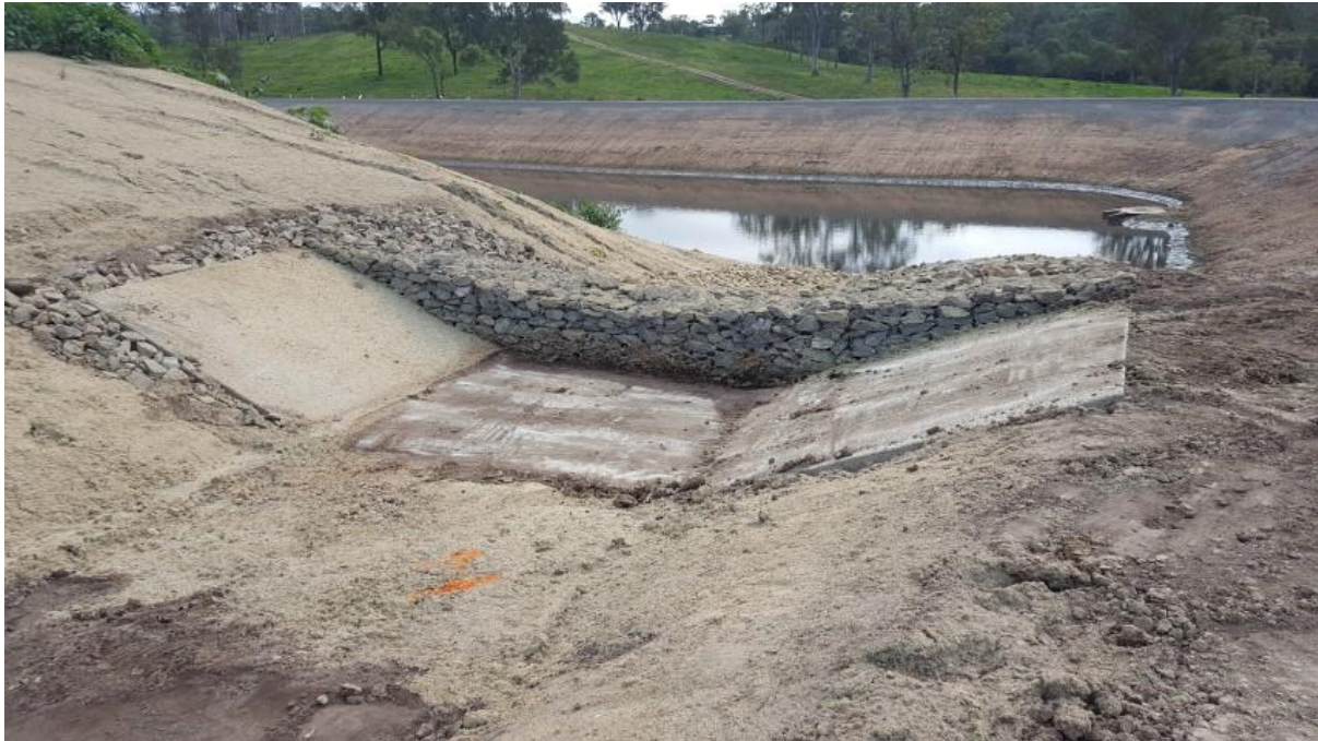
Figure 5: Rock gabion installed at the Western Contaminated Pond inlet.
