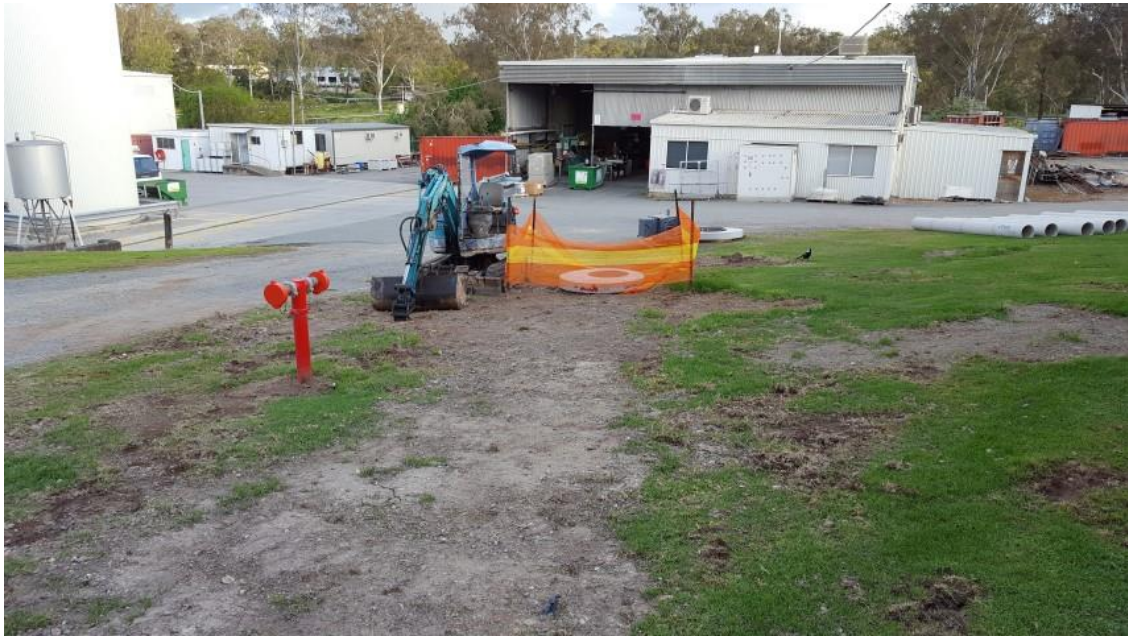
Figure 3 Stormwater Drainage Upgrade Progress
