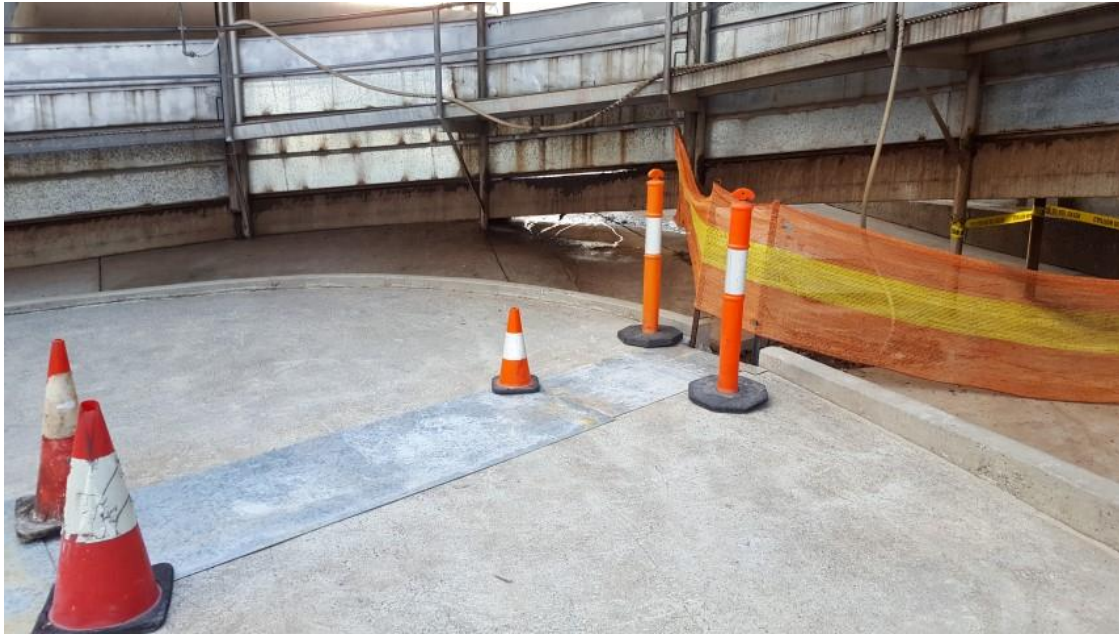
Figure 4 Stormwater drainage upgrade progress
