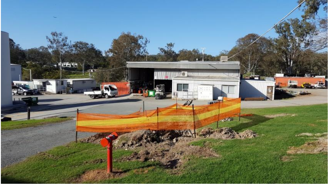
Figure 2 Stormwater Drainage Upgrade Progress
