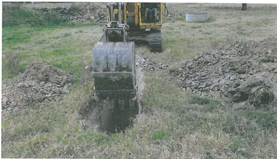
Figure 5: Example photo of test pit progress.
