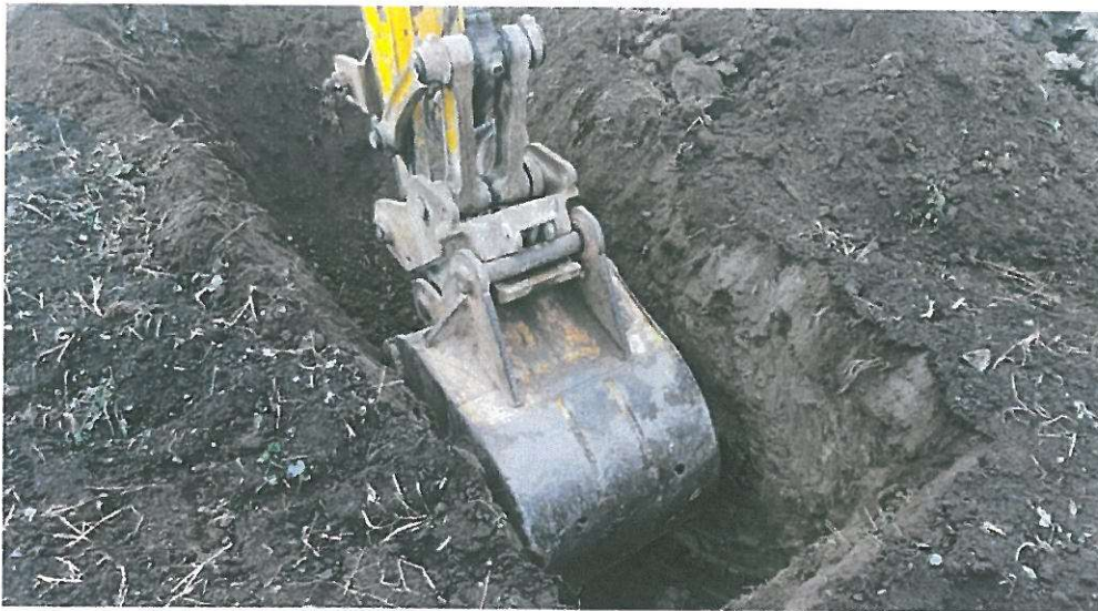
Figure 4: Example photo of test pit progress.
