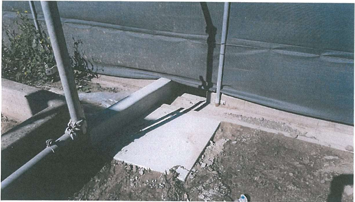
Figure 11. AFTER Western side of the covered yard including bund wall.
