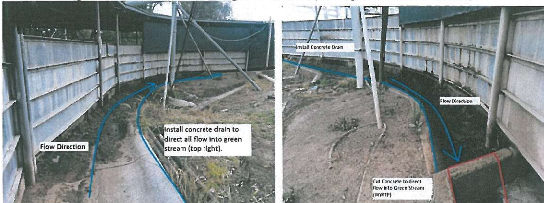
Figure 8 BEFORE. Proposed concrete drainage to be installed and direct potentially contaminated streams to the wastewater treatment system.
