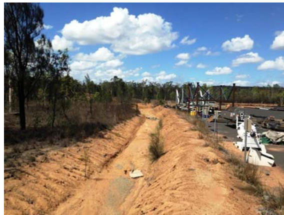
Figure 8 – NW Clean water Drain.
