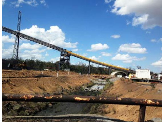
Figure 9 – Clean water drain with rock checks.
