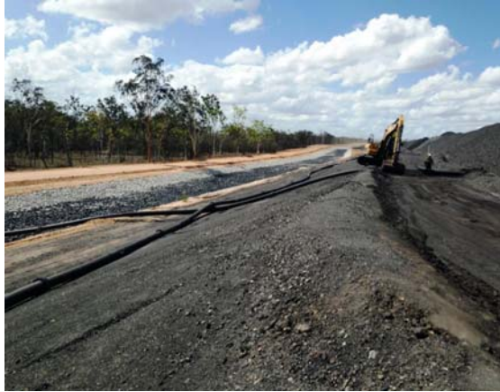
Figure 3 – Western Toe Drain
