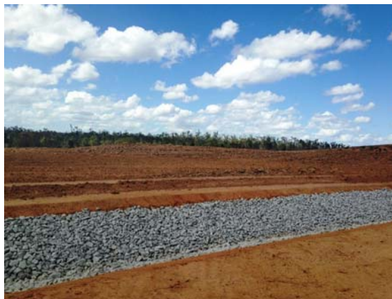
Figure 2 – Co-Disposal Topsoil stock pile Ripped and Seed
