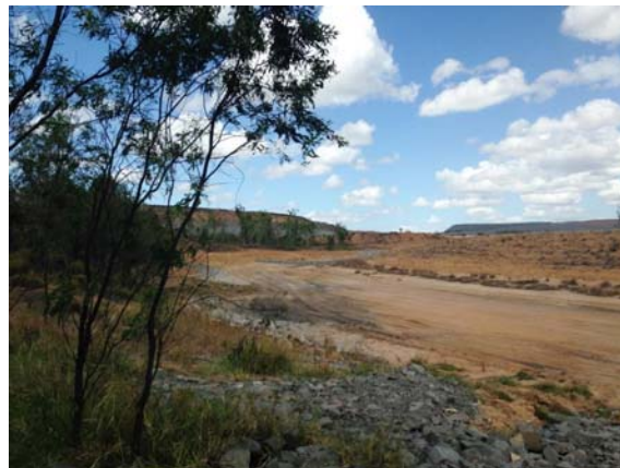
Figure 6 – Rock Checks in South Arm Diversion.
