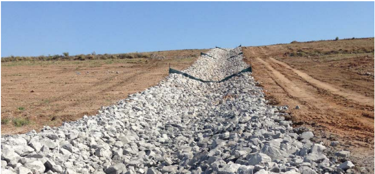
Figure 2: Rock-lined Down Drain with Sediment Fences
