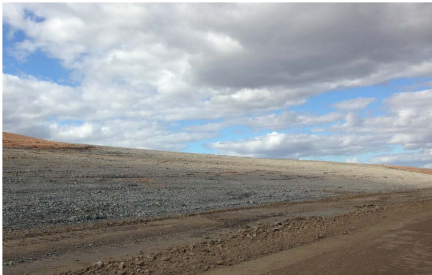
Figure 10: Radio Hill Reshaped and Permian Capped Landform - Lower Tier (East)
