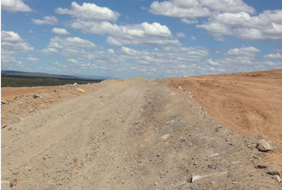
Figure 1: Contour Banks
