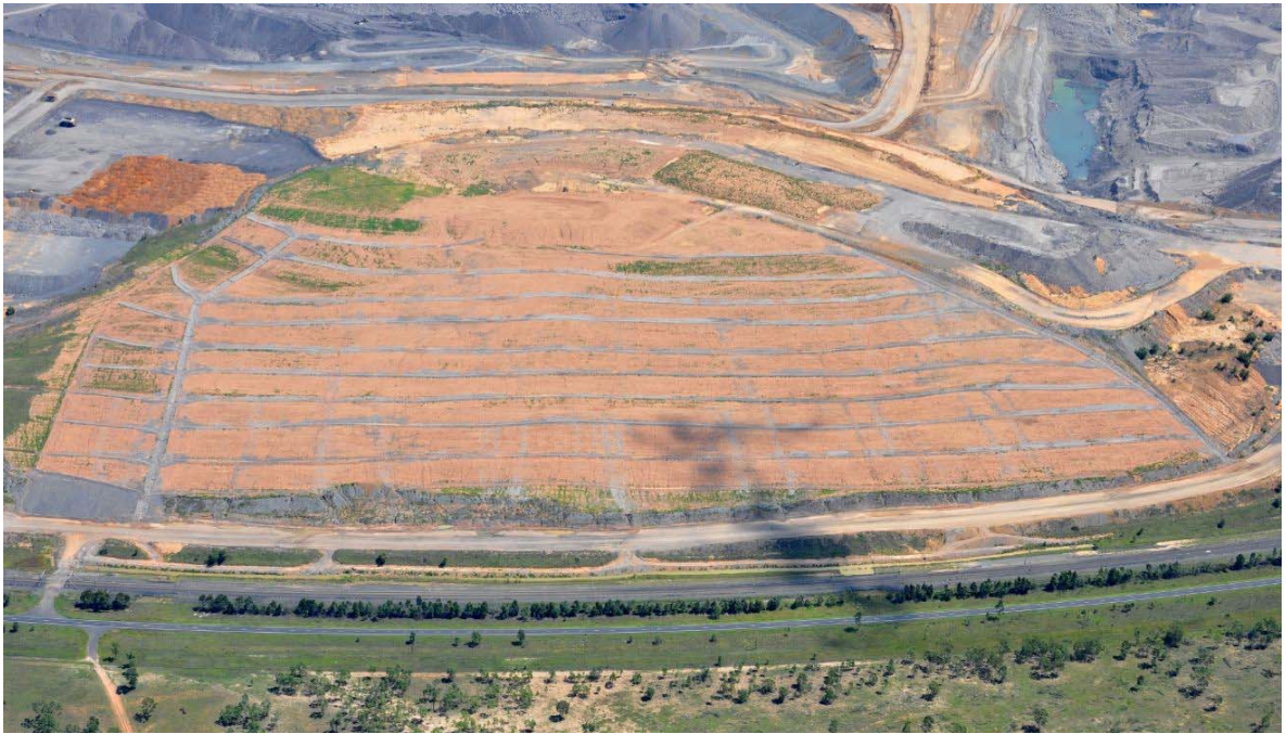
Figure 3: Remediated F-Dump Landform
