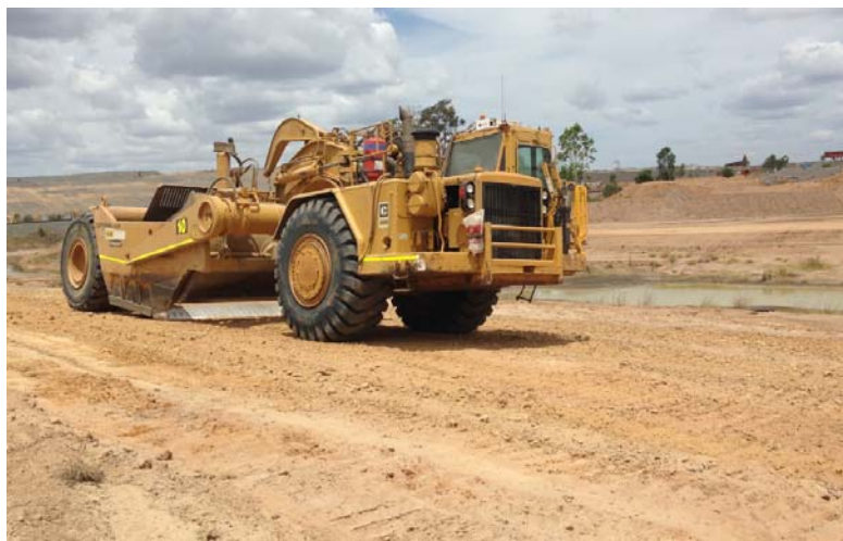
Figure 4: Scraper conducting topsoiling Thirty Mile Creek South Arm Diversion banks
