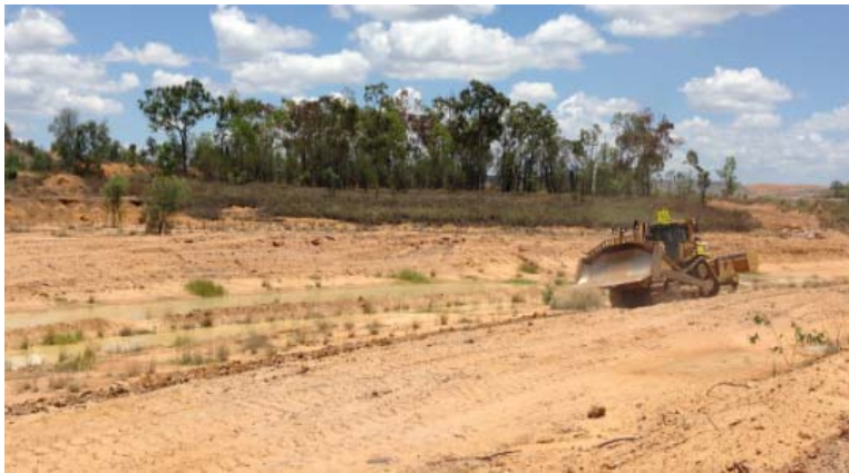
Figure 5: D8T Dozer with drum seeder undertaking combined ripping and seeding activities
