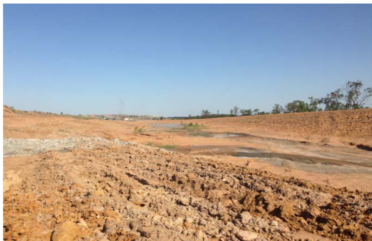
Figure 7: Ripped and Seeded Thirty Mile Creek South Arm Diversion Bank (downstream)
