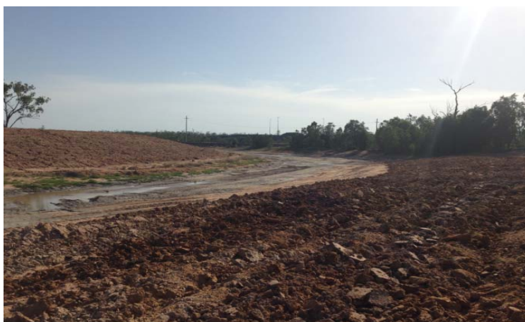
Figure 6: Ripped and Seeded Thirty Mile Creek South Arm Diversion Banks (upstream)
