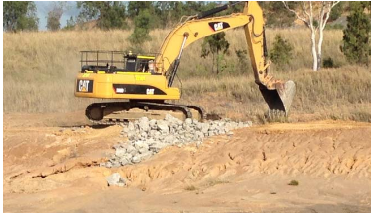
Figure 1: Filling of erosion scours with competent Permian material
