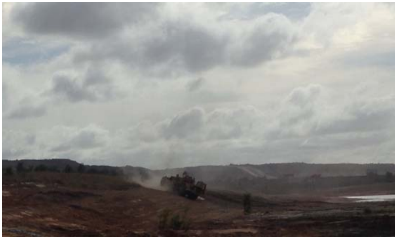
Figure 3: Scraper conducting topsoiling on Thirty Mile Creek South Arm Diversion banks
