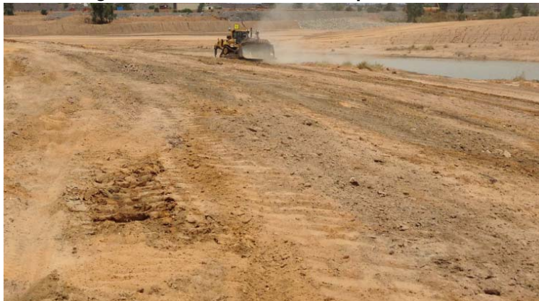
Figure 2: Removal of Erosion Scours
