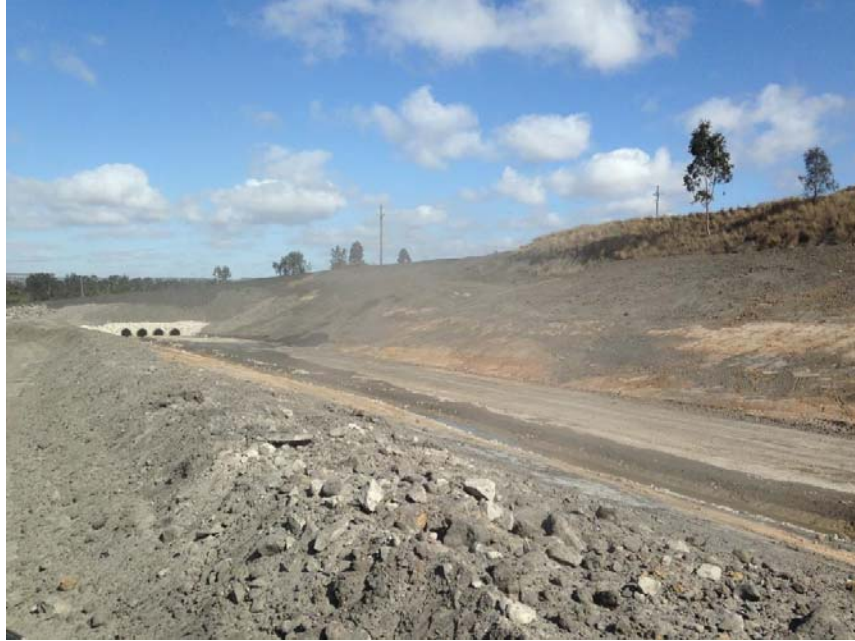
Plate 5 – Eastern Toe Drain: Tie into Return Water Dam
