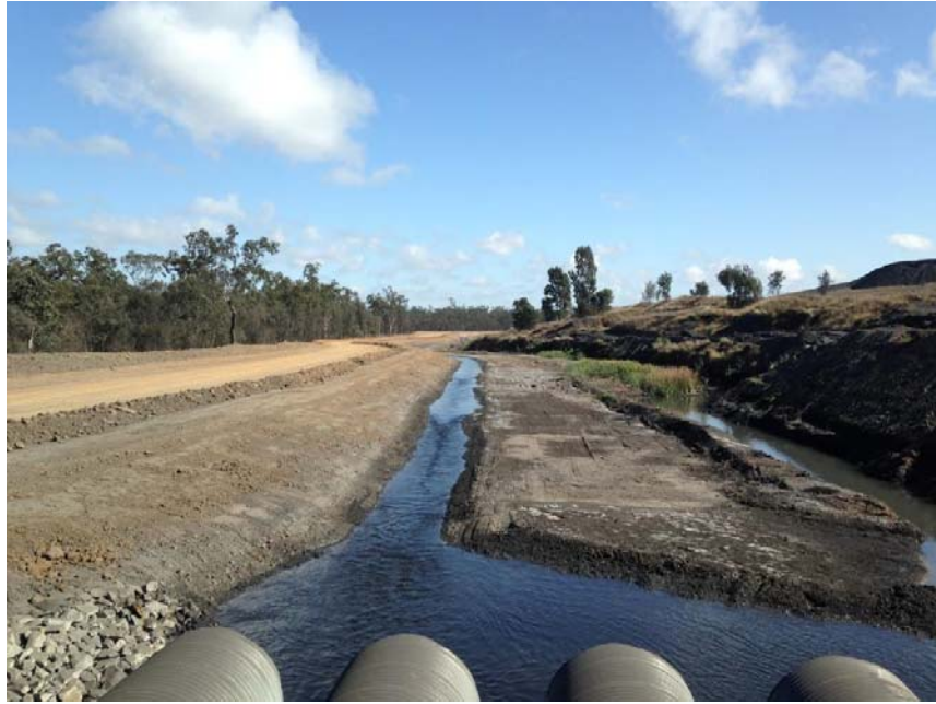
Plate 1 – Western Toe Drain: Entry to Return Water Dam to First Bend
