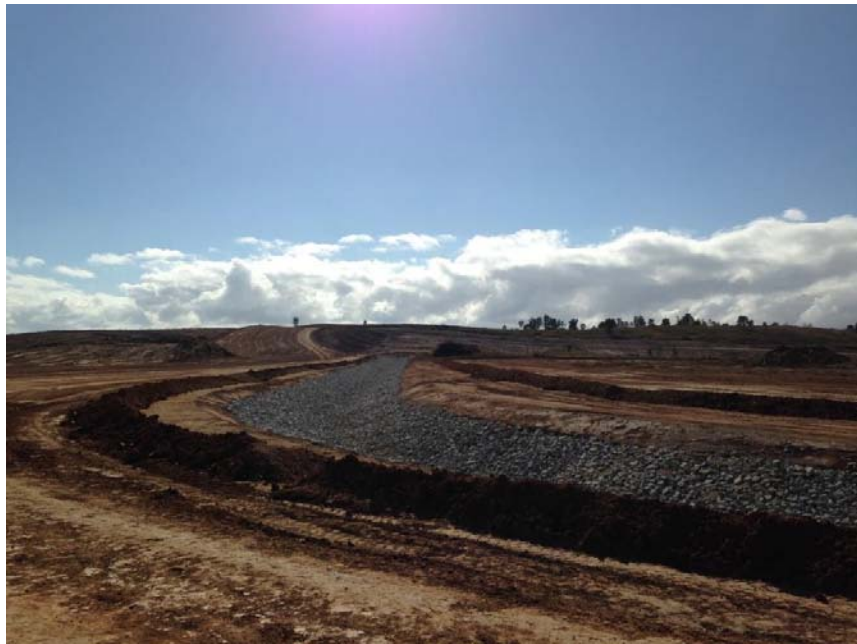
Plate 4 –Western Toe Drain; Tie into existing landform
