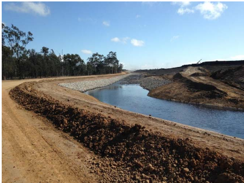
Plate 2 – Western Toe Drain First Bend to end of Cell 1
