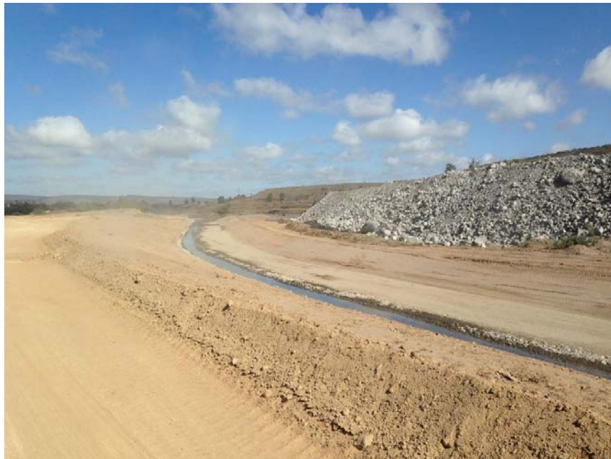
Plate 6 – Eastern Toe Drain; First Corner to Tie into RWD
