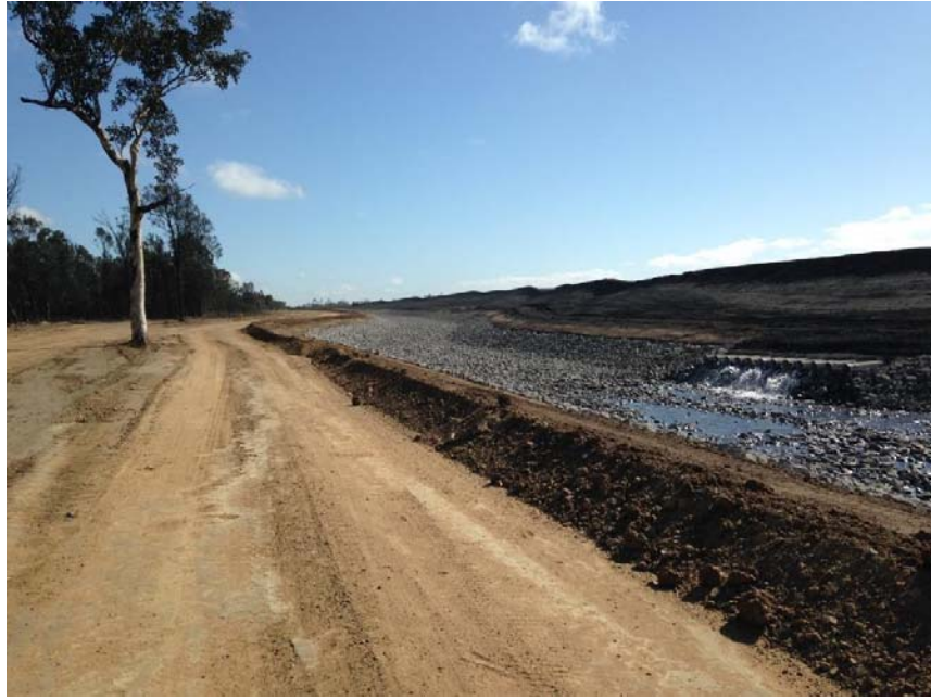
Plate 3 –Western Toe Drain; End of Cell1 to End of Cell 2
