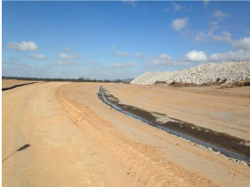
Plate 7 – Eastern Toe Drain; Second Corner to First Corner
