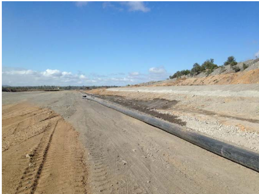
Plate 8 – Eastern Toe Drain; Start to Second Corner
