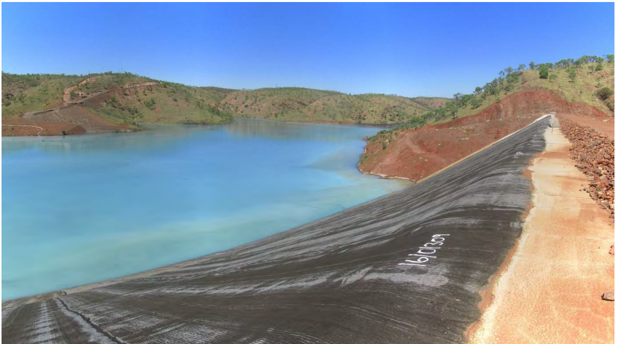
Figure 24 Coletanche Installed in Hot Climate with no wrinkling evident
