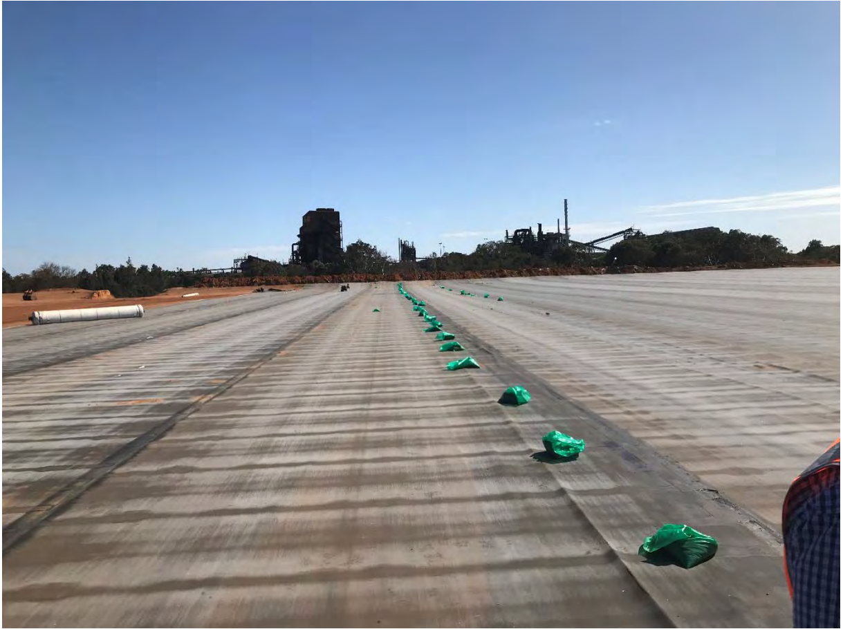
Figure 23 Coletanche SC1 installed in WA
