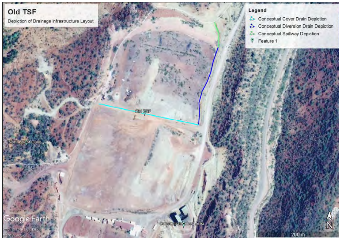
Figure 1 Old TSF drainage structure's layout (Google Earth, 2018)
