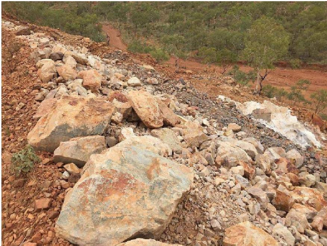
Photo 16 Eastern Embankment of HLEP #2 near BH11
