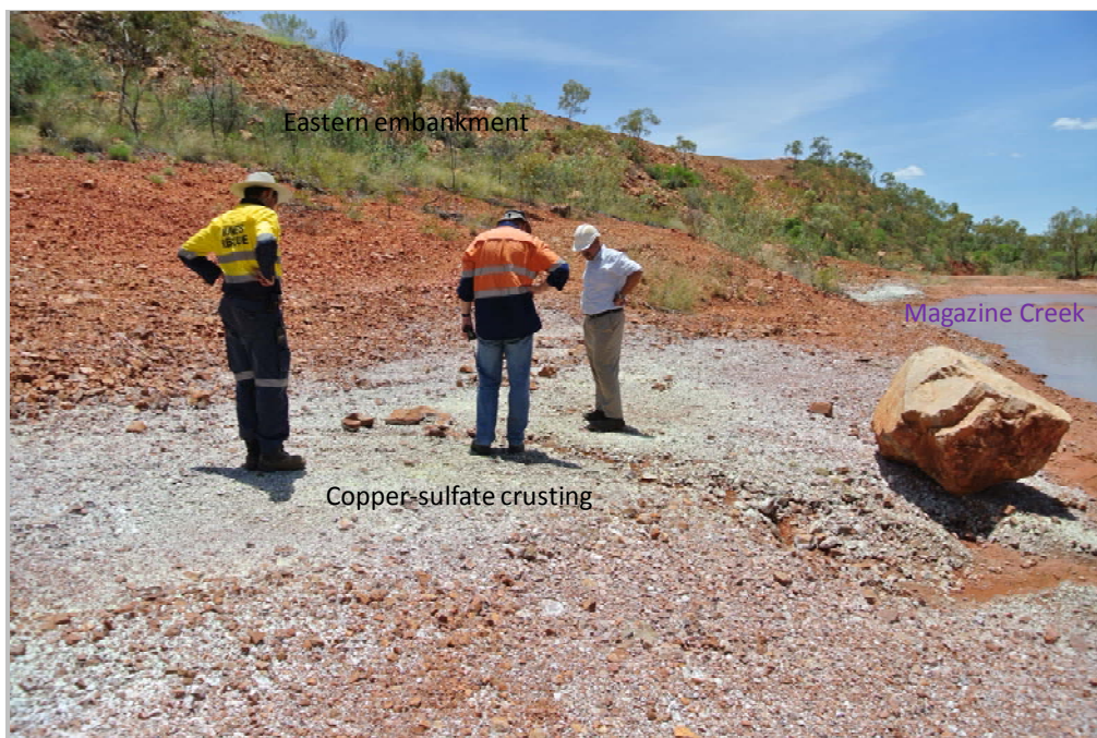
Figure 2.4 Heap leach pad number 2 eastern embankment
