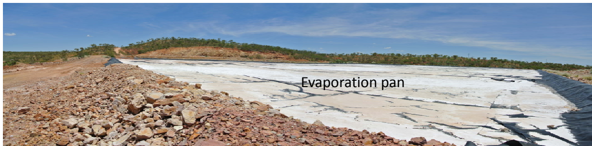
Figure 2.5 Heap leach pad number 2 evaporation pan
