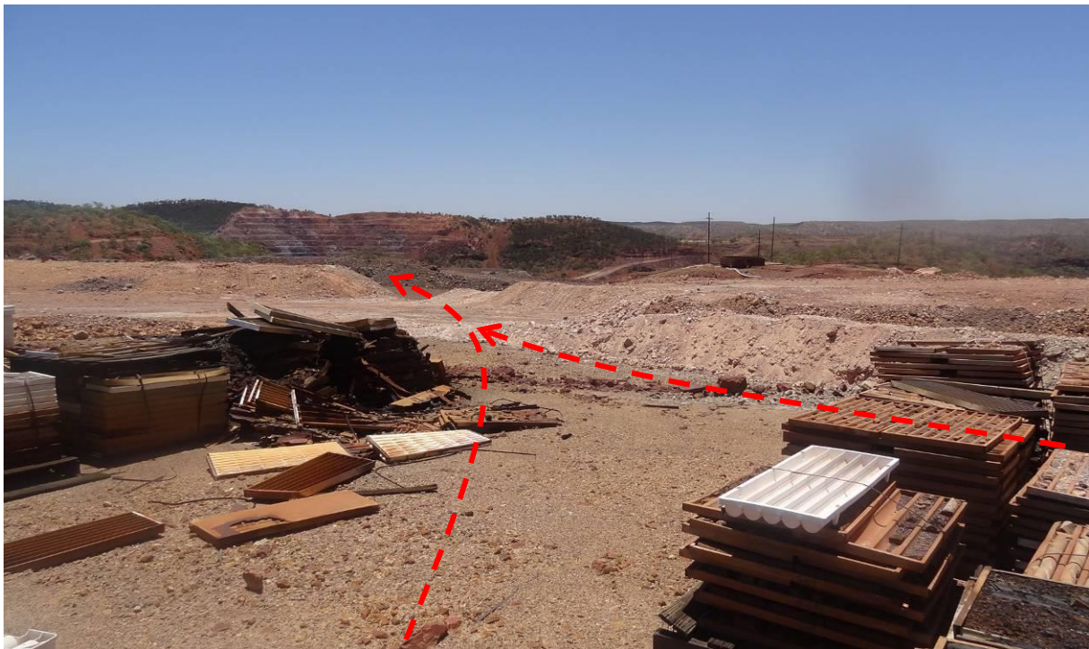
Earthworks to reduce contaminated water from Heap Leach #1 drains to Pit and not Magazine Creek.
