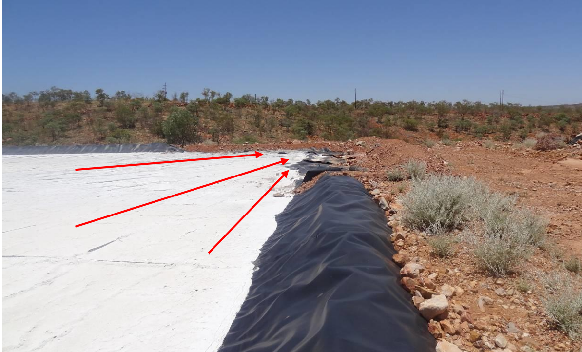
Excavation of Heap Leach #2 Evaporation Pond's spillway, ensuring facility cannot pool water.
