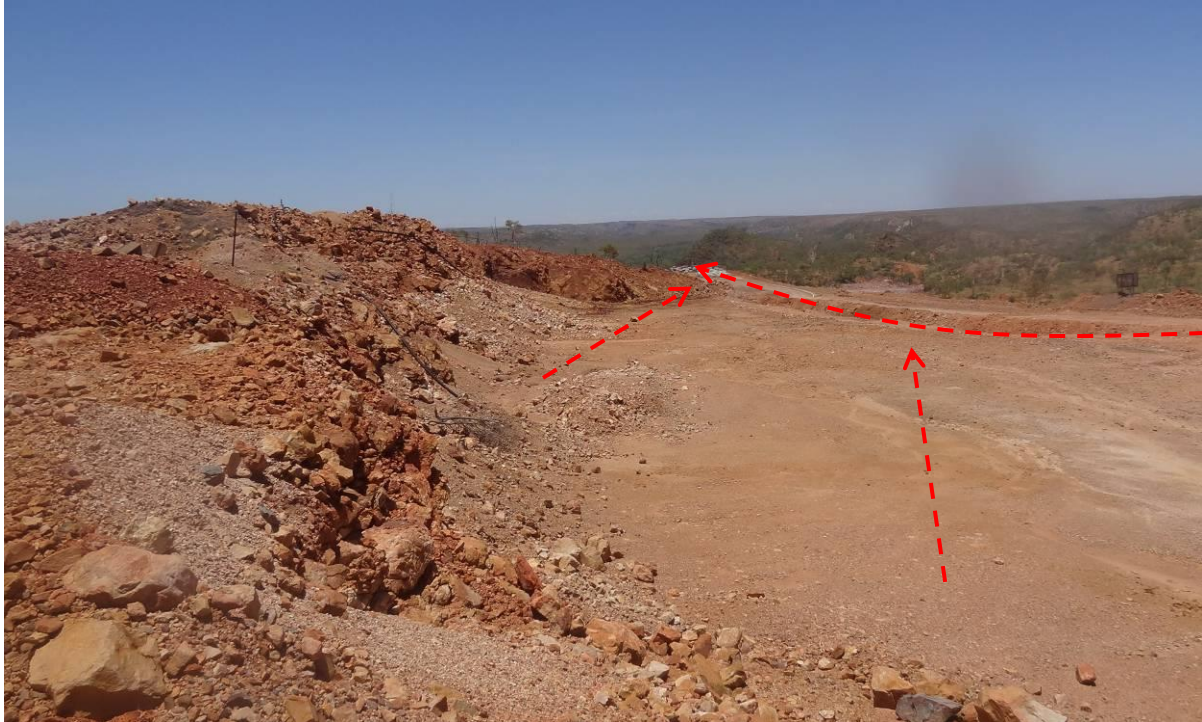
Earthworks to ensure contaminated water from Mammoth Hill drains to pit and not Magazine Creek.
