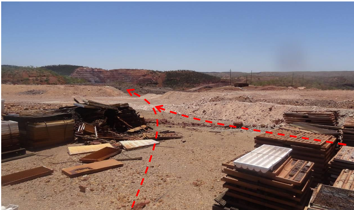
Earthworks to ensure contaminated water from Heap Leach #1 drains to Pit and not Magazine Creek.
