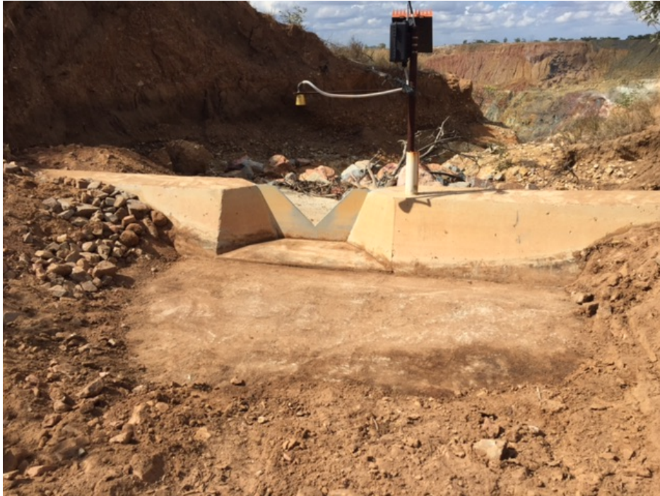
Figure 4: Maintenance of SF1 stream flow gauge
