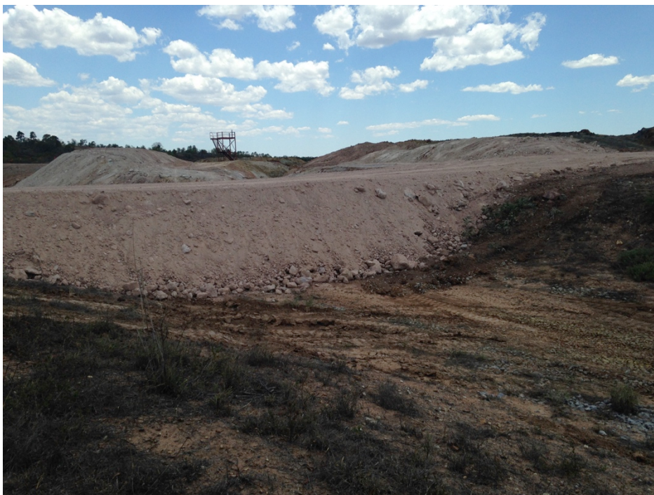
Figure 2: Diversion bund facing towards Highway Reward pit
