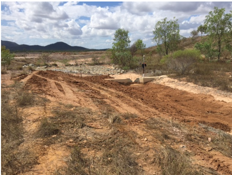
Figure 3: Maintenance of SF2 stream flow gauge
