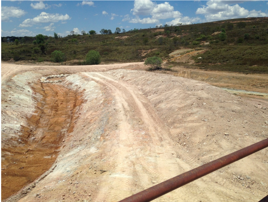
Figure 1: Diversion drain facing towards Highway Waste Rock Dump
