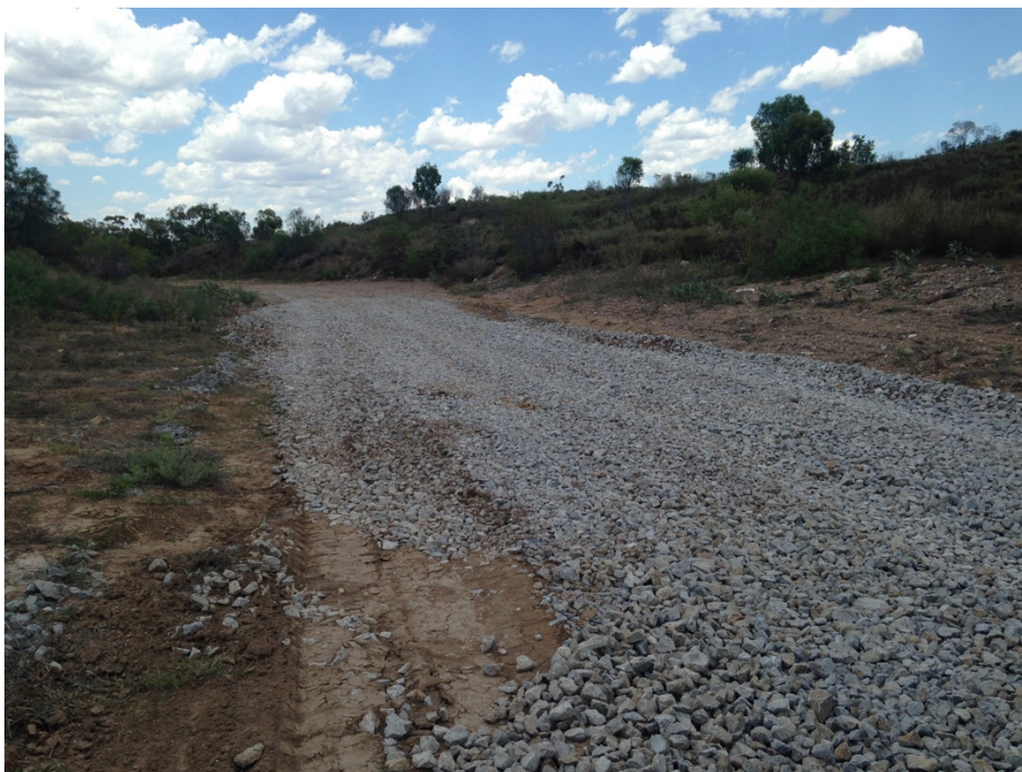
Figure 5: Maintenance of lime rock in main drain
