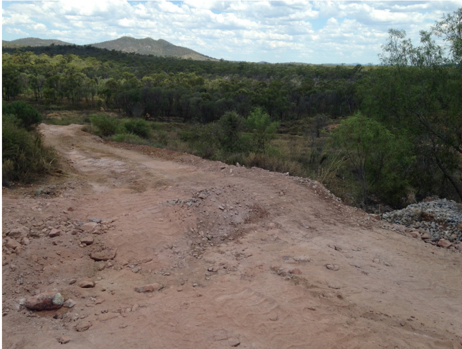
Figure 6: Maintenance of access tracks
