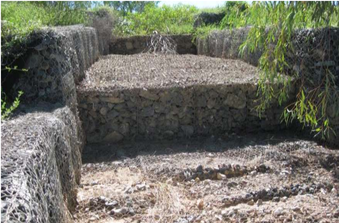
Drop structures in main drain, rock filled gabions
