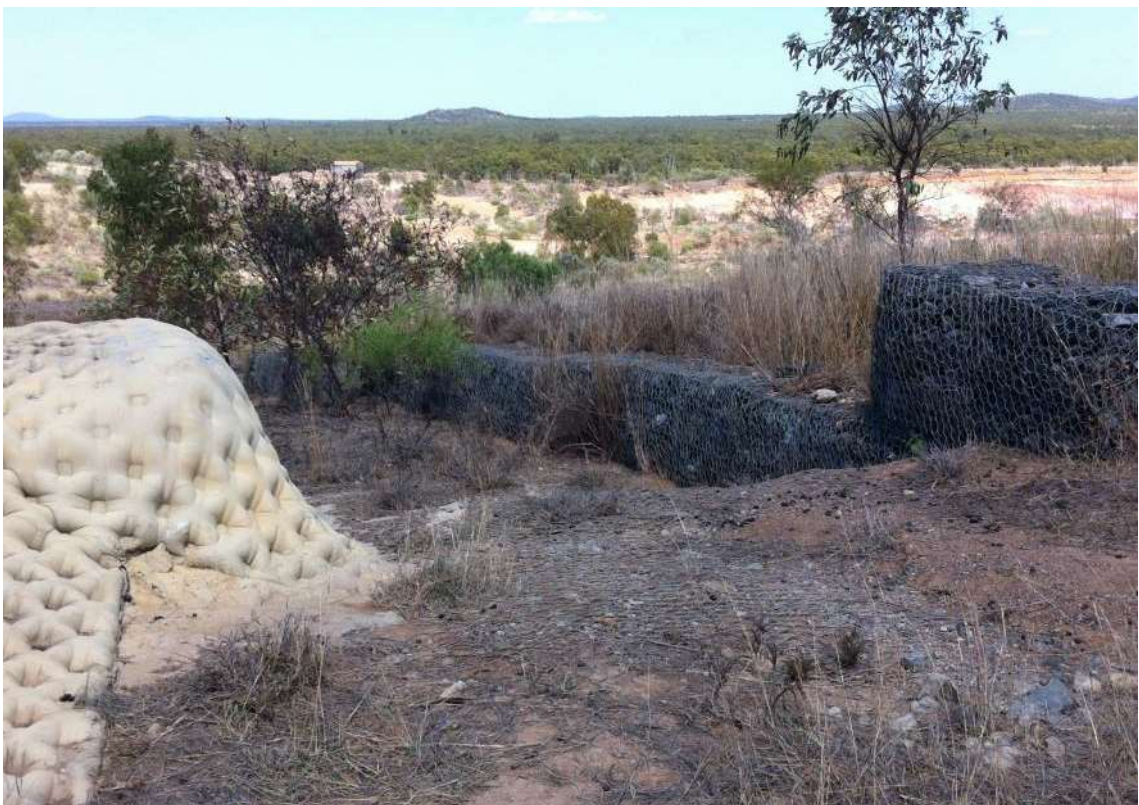
Entry to main drain, recent revetment mattress protection
