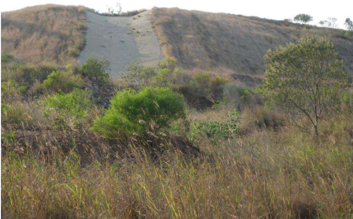
Grout filled revetment mattress, southeast Reward dump drop structure
