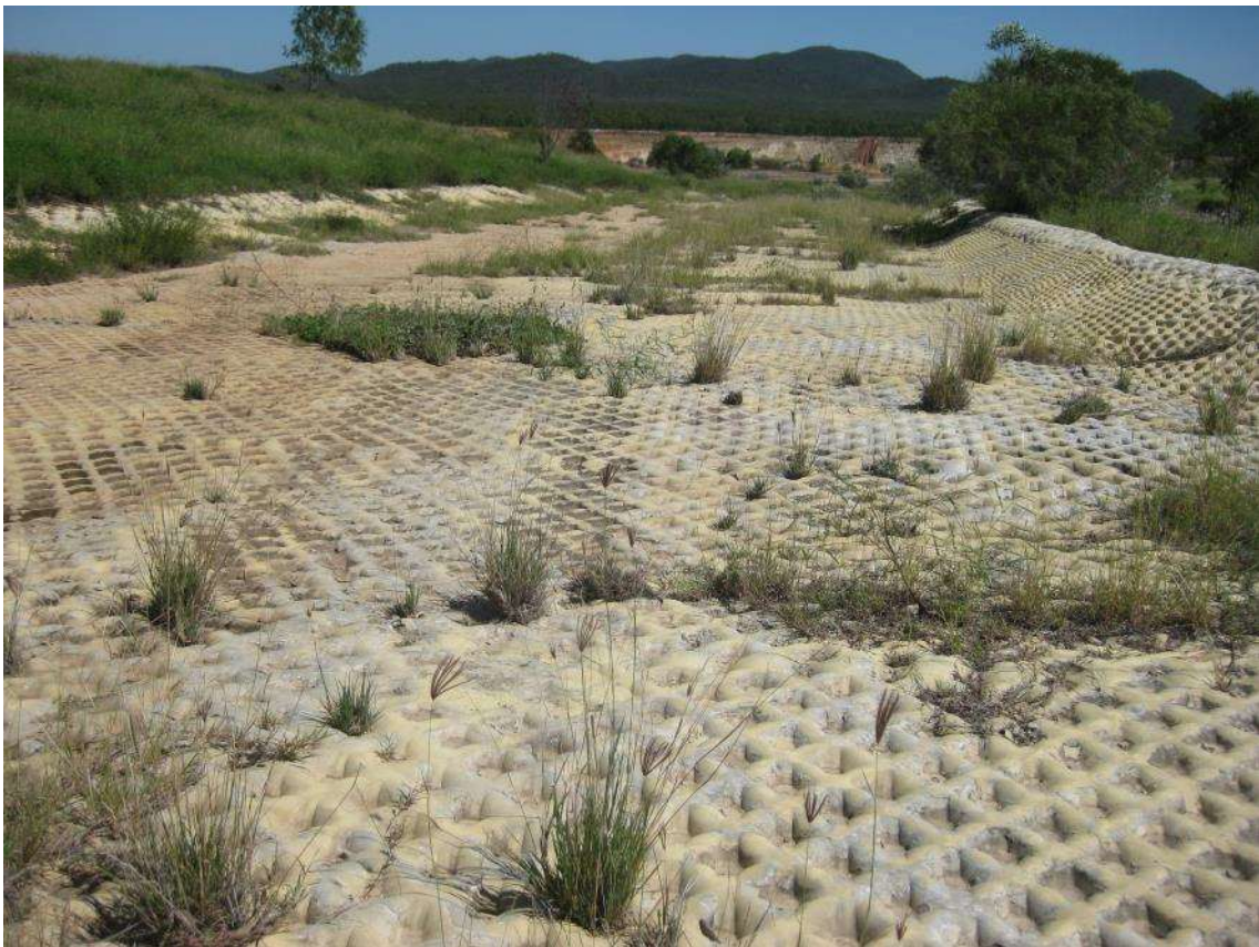
Grout filled revetment mattress, top end main drain.
