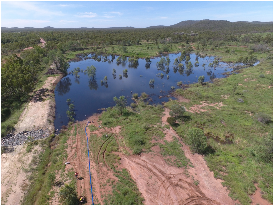
Figure 2: Pumping activities at the old TSF evaporation pond.
