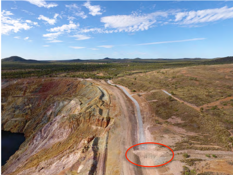
Figure 4: Installation of diversion bund to direct flow to the main pit (circled in red).
