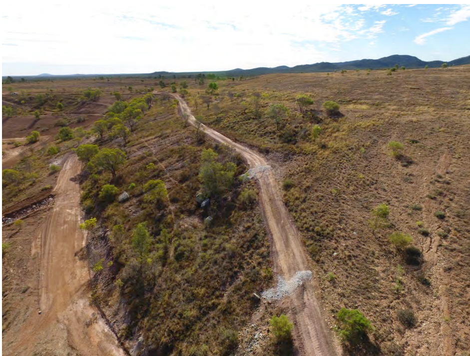
Figure 6: Evidence of erosion protection measure restoration works to eroded areas.
