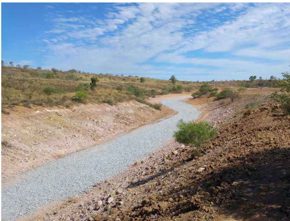
Figure 2: Main drain with lime rock armouring.
