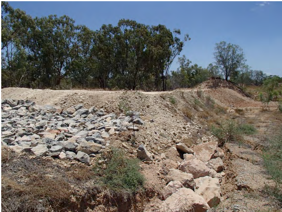
Figure 3: Completed reprofiling and repair works to western storage.
