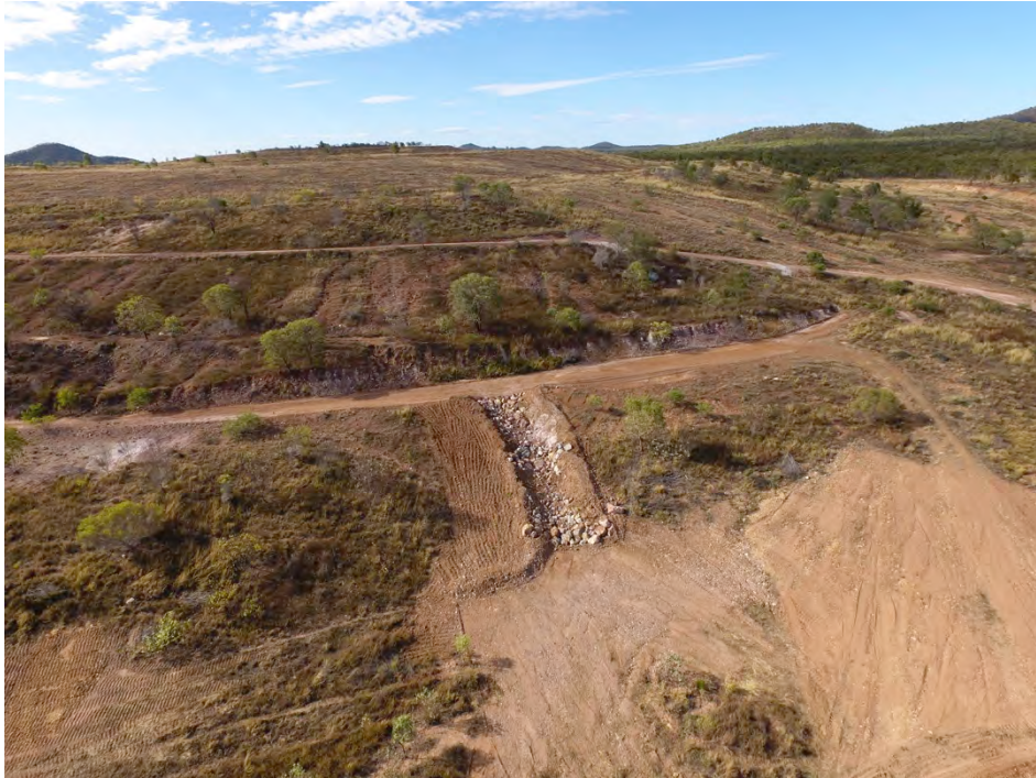
Figure 5: Evidence of erosion protection measure restoration works to eroded areas.
