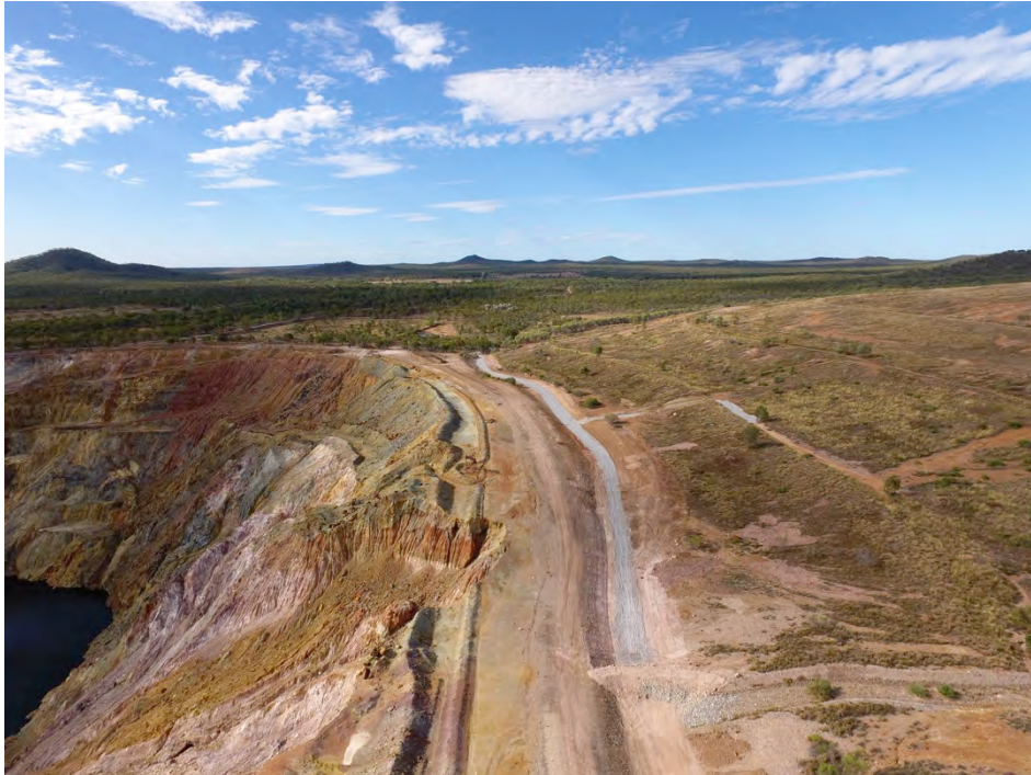
Figure 1: Elevated view of main drain with lime rock armouring.
