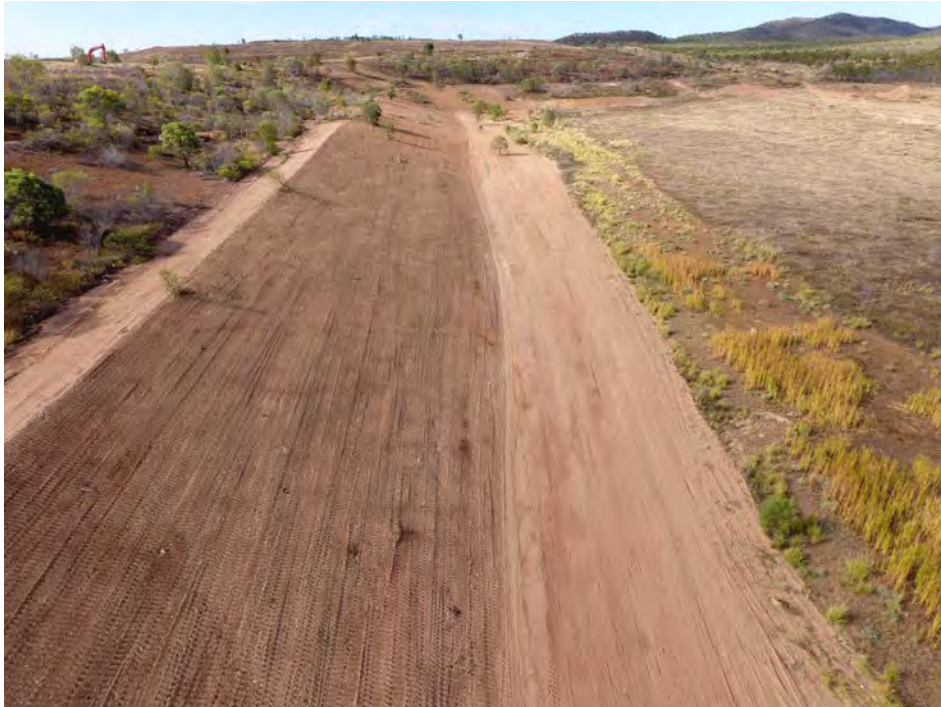
Figure 7: Evidence of restoration works to eastern batter of dump known as Reward.
