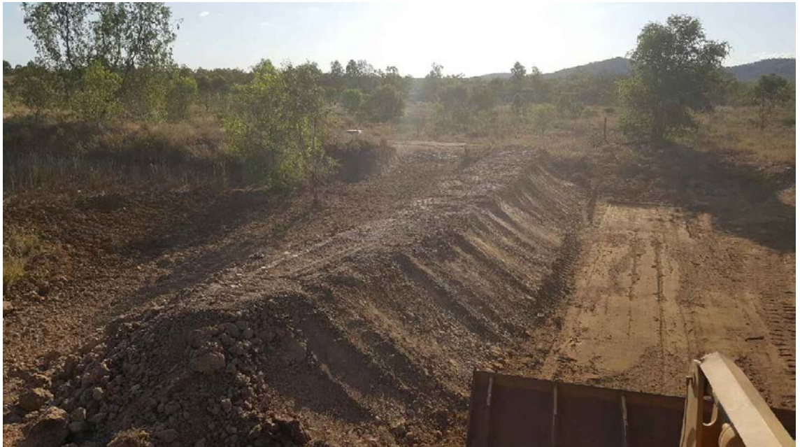
Figure 3: Completion of bund installation to prevent water release offsite towards SW6.
