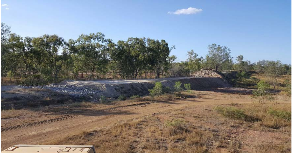
Figure 4: Completion of earthworks to re-instate bund on eastern perimeter of historic tailings storage.
