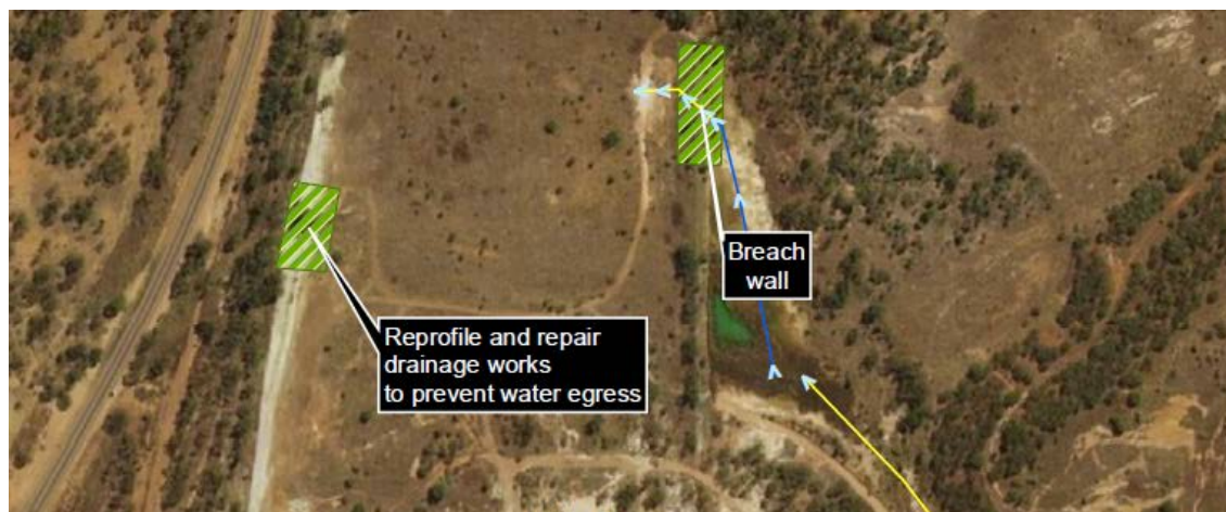
Figure 1: Representation of earthworks completed by 1 November 2016.
