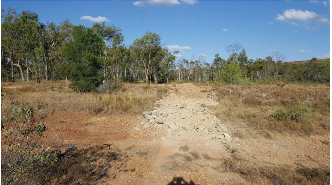
Figure 2: Completion of breach and lime rock armouring from main drainage to historic tailings storage.
