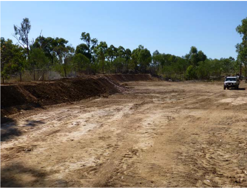
Plate 4 Diversion bund Western flow path
