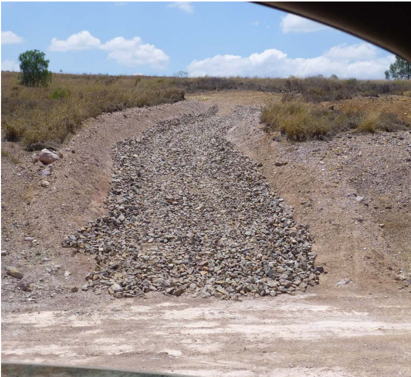
Plate 10 S drop Structure
