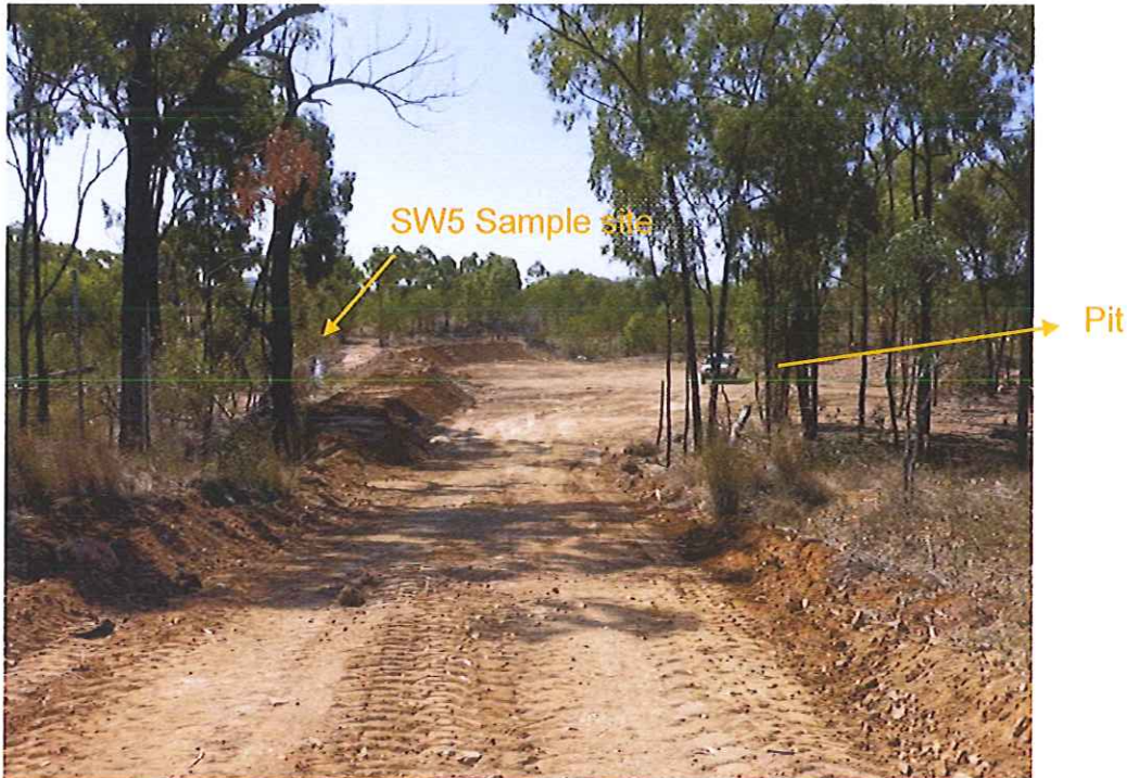
Plate 1 Diversion bund western side of lease
