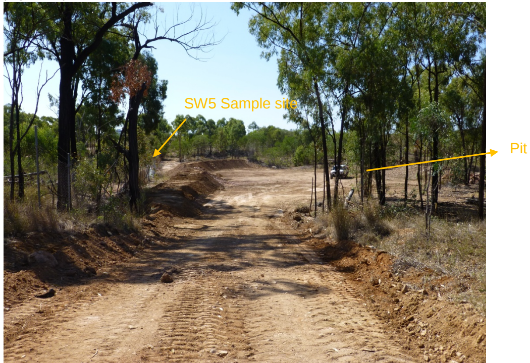
Figure 15: Diversion bund on western side of lease
