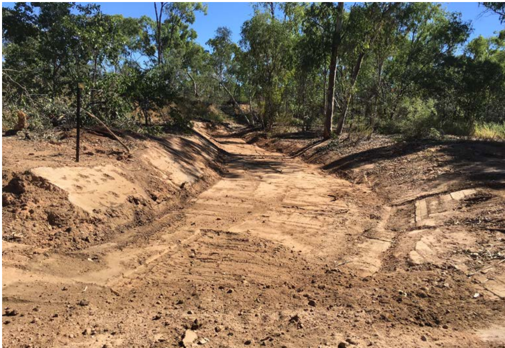
Figure 2: Completion of earthworks at SS7
