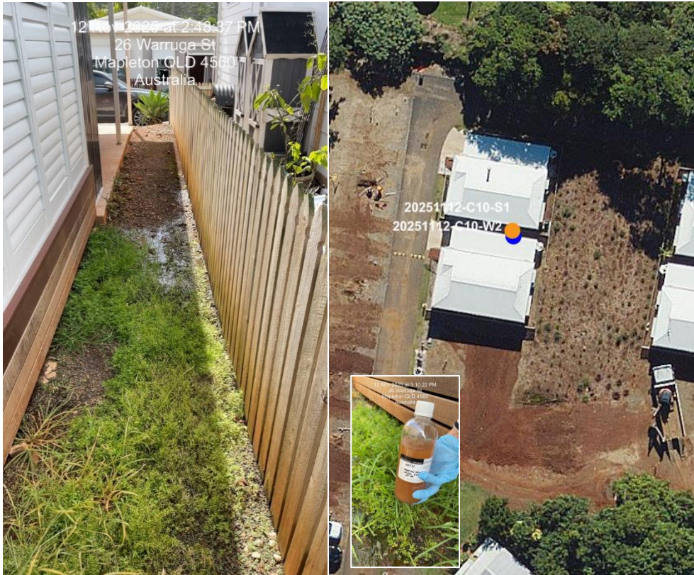
Figure 2 – Effluent ponding within backyard of cabin 10 residence and location of sample W2 and S1
