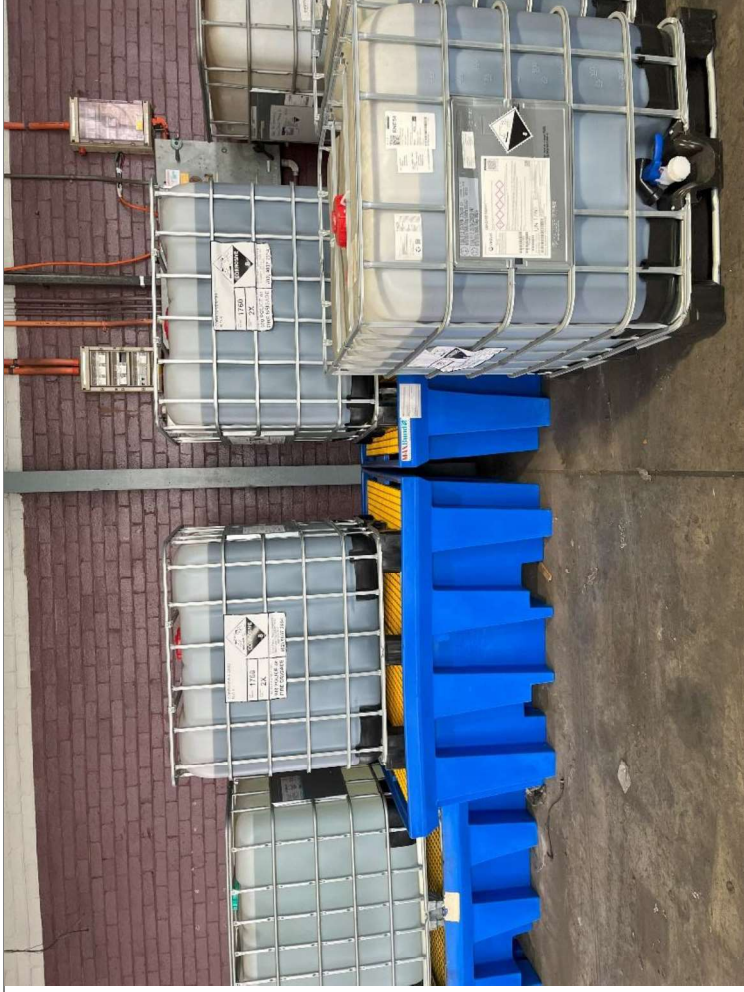
Photo 9: Bulk Chemical Storage building. Chemicals stored contravention to EA conditions, absence of secondary bunding to prevent surface flow of spilled chemicals. Image captured by the departmental officers, 3 January 2025.
