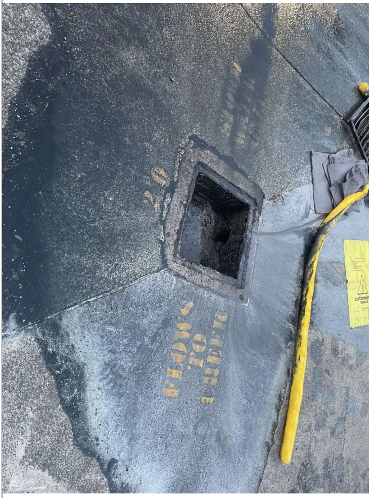
Photo 6: Stormwater drain to the west southwest of the Bulk Chemical Storage building. Image captured by the QFD officers, 31 December 2024.
