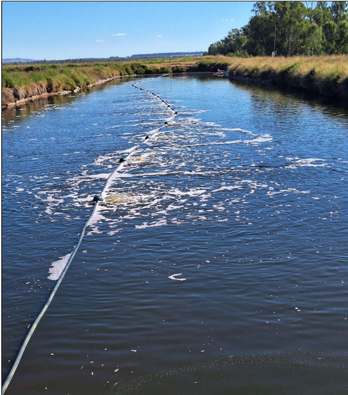
Figure 2: Photograph of irrigation lagoon with new aeration system installed and operating. Photo taken on the 24/06/2026.
