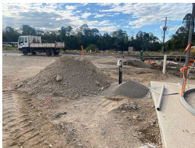
Figure 2 – Underground electrical works progressing
