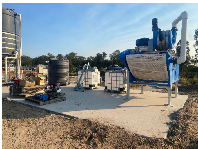
Figure 2 - Installation of filtration system continuing
