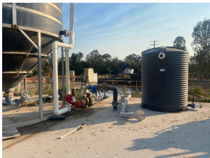
Figure 1 - Storage and settling tanks installation continuing
