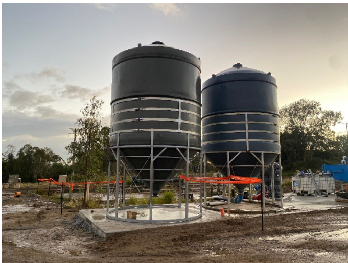
Figure 1 - Storage and settling tanks installation commenced
