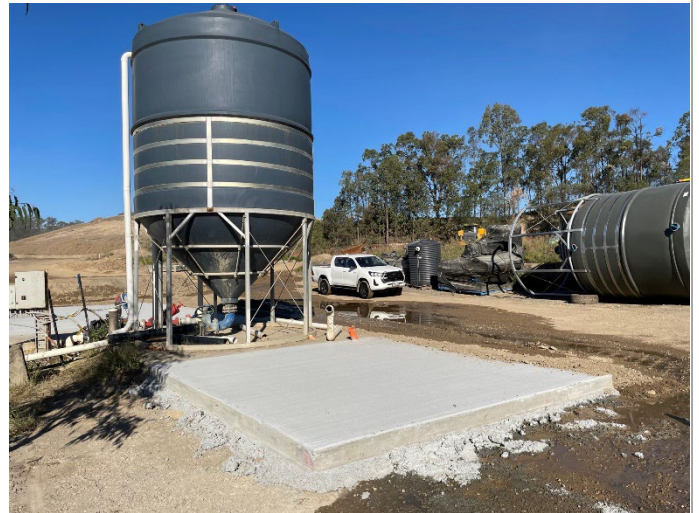
Figure 1 – Civil works for wheel wash ancillary structures ongoing.
