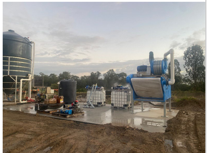
Figure 2 - Installation of filtration system commenced
