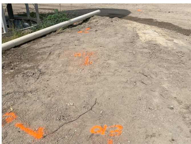
Figure 5 – Example of underground services survey in preparation for civil works at wheel wash
