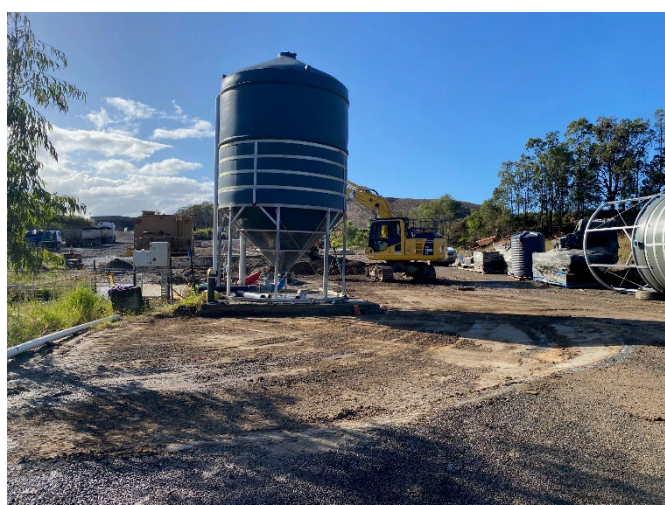
Figure 6 - Commencement of civil works for wheel wash ancillary structures
